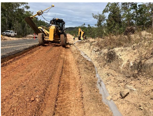
Road widening in cutting
