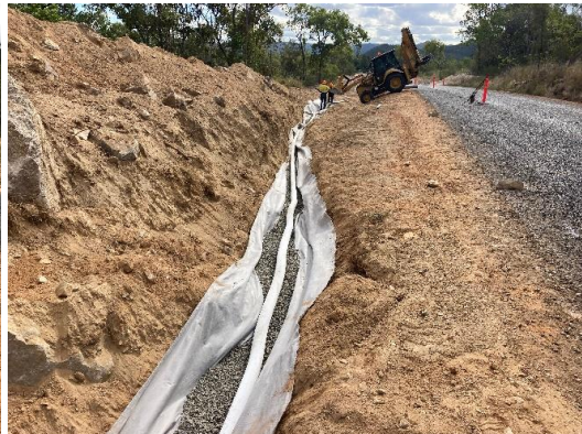
Subsoil drain installation
