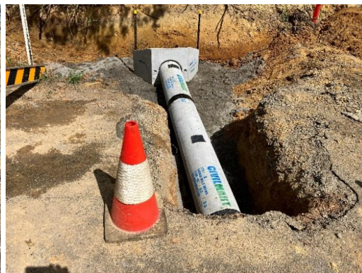
375Ø RCP extension (Ch 9425)
