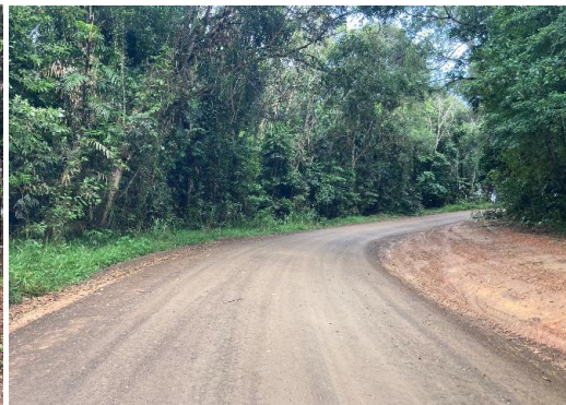
Black Mountain Road Gravel Re-Sheet
