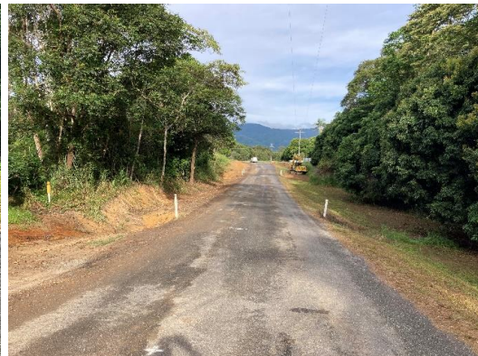
Euluma Creek Road After Clear and Grubbing
