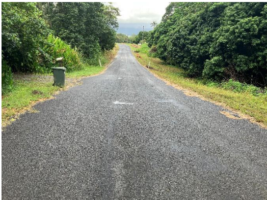
Euluma Creek Road Before Clearing and Grubbing
