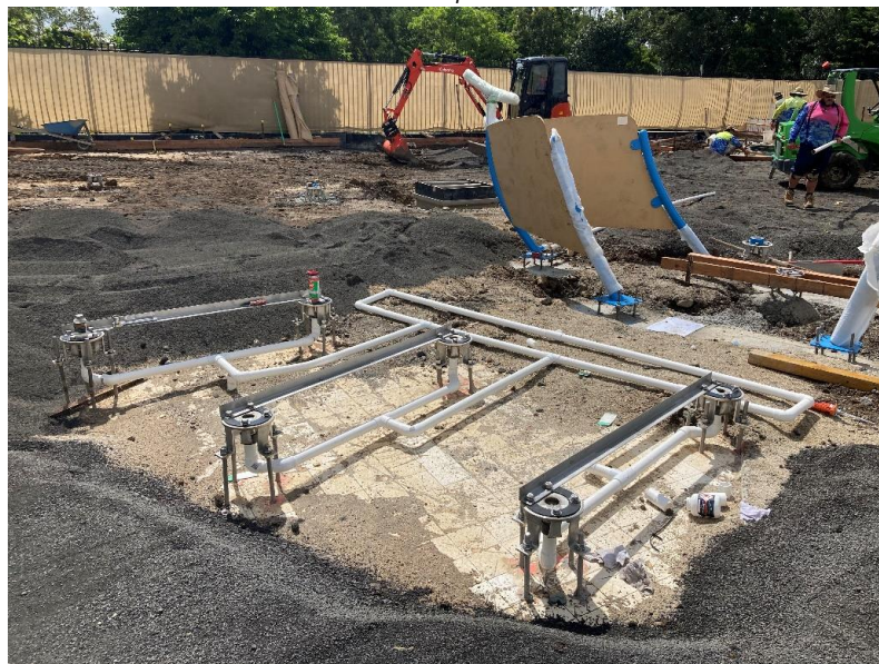
Plumbing and Play Equipment Preparation
