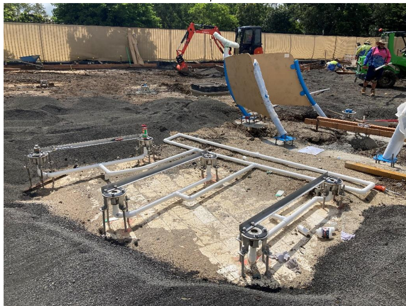
Plumbing and Play Equipment Preparation
