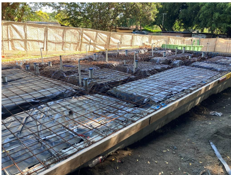
Riverside Caravan Park Base Construction
