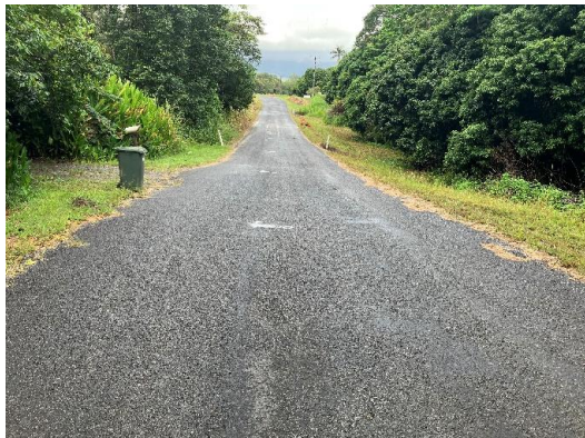
Euluma Creek Road Before Clearing and Grubbing
