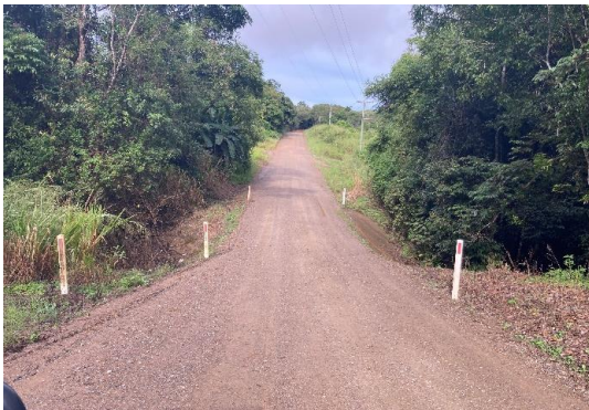
Black Mountain Road Gravel Re-Sheet
