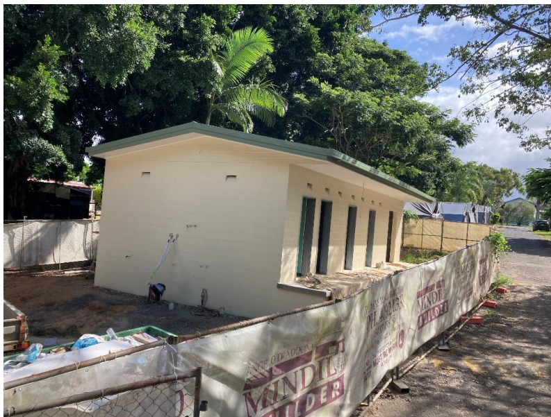
Riverside Caravan Park Amenities External Paint
