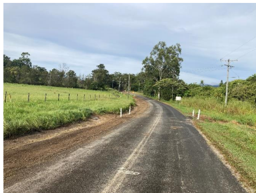
Euluma Creek Road Drain Reestablishment
