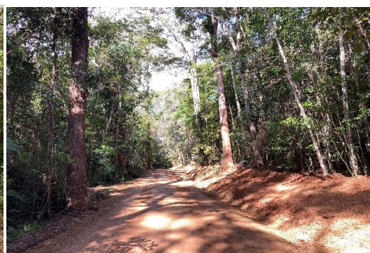
Bump Track Gravel Re-Sheet
