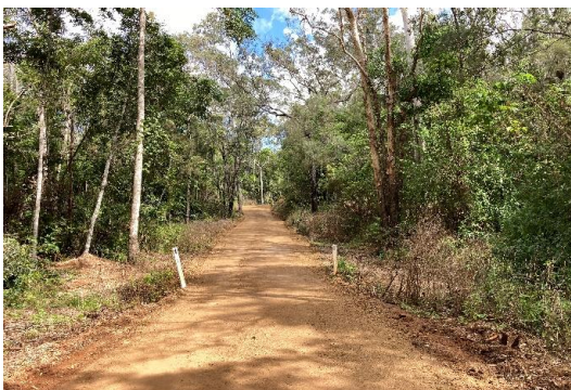
Riley Road Gravel Re-Sheet
