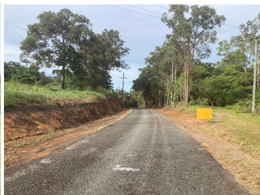
Euluma Creek Road Batter Cleaning
