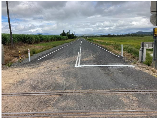
Borzi Road – Project Start
