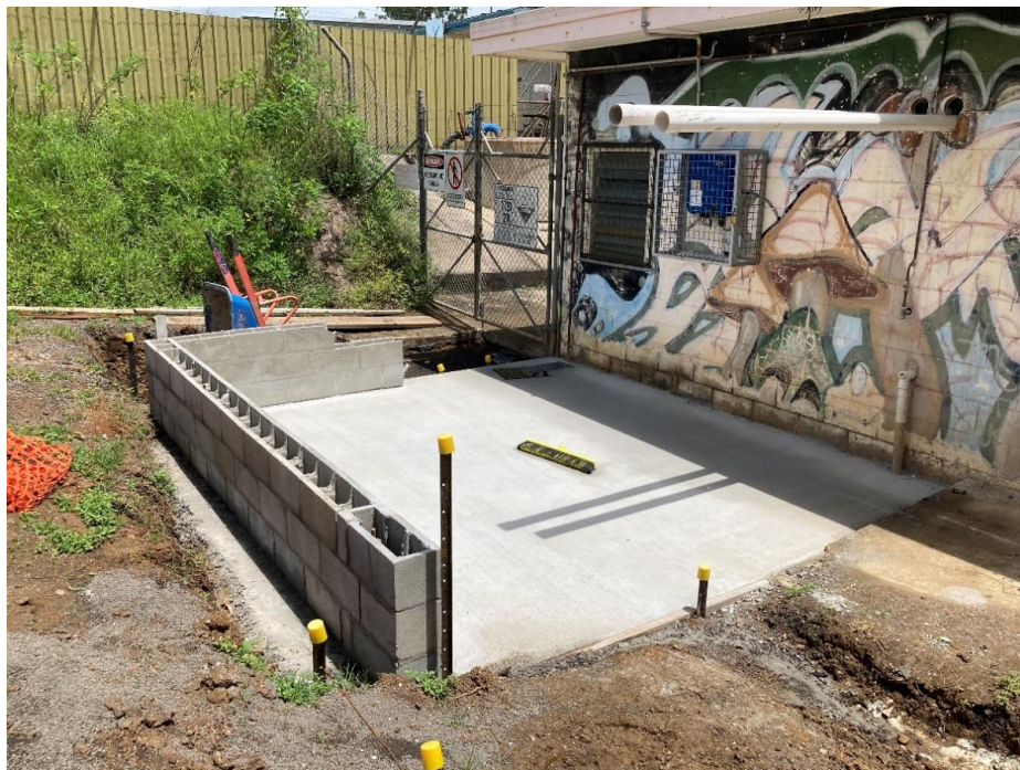
Site preparation for heat pump installation
