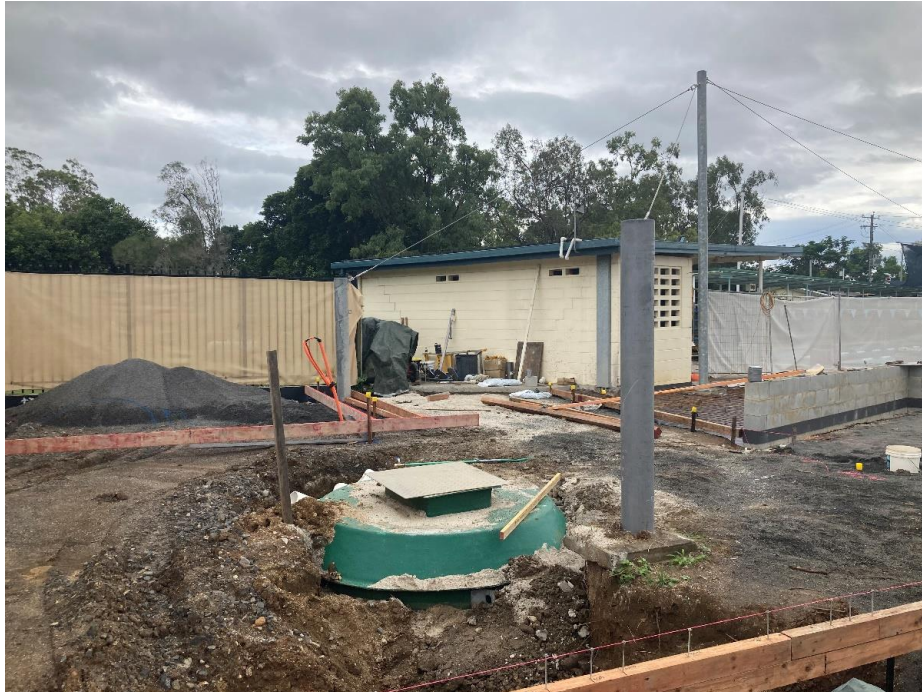
Installation of Balance Tank for Splash Park
