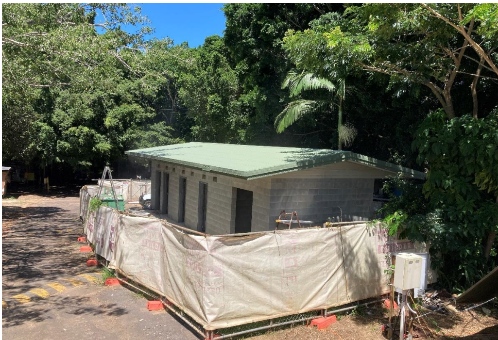
Riverside Caravan Park New Amenities Block – completion of walls and roof
