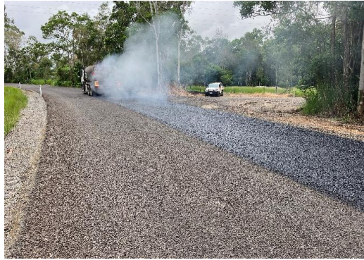
Binder application second coat 10mm seal - Section B
