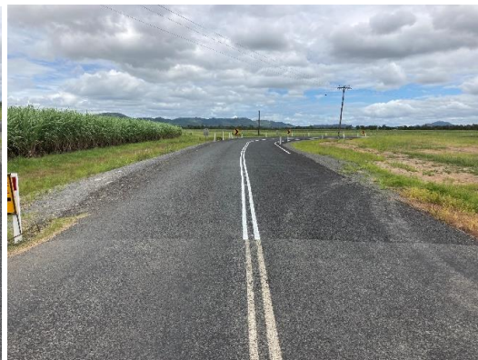
Borzi Road - Project End
