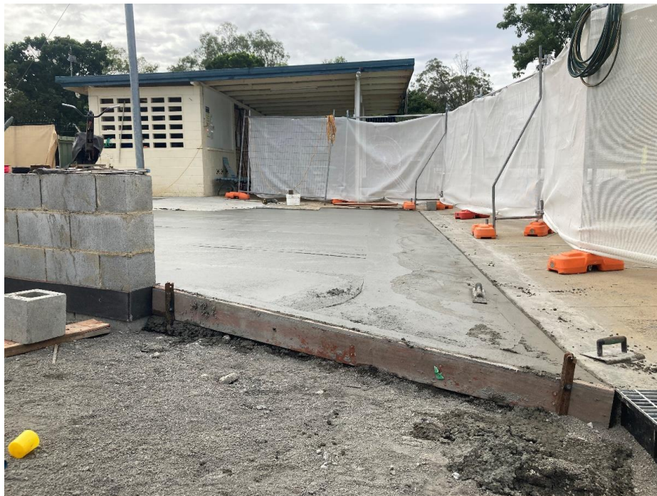
Existing pavers replaced with new concrete between old clubhouse, 50m pool and new Splash Park
