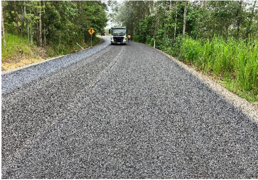
Second coat 10mm seal - Section B
