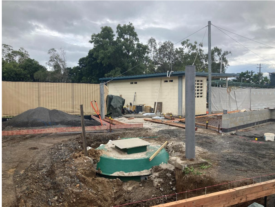
Installation of Balance Tank for Splash Park
