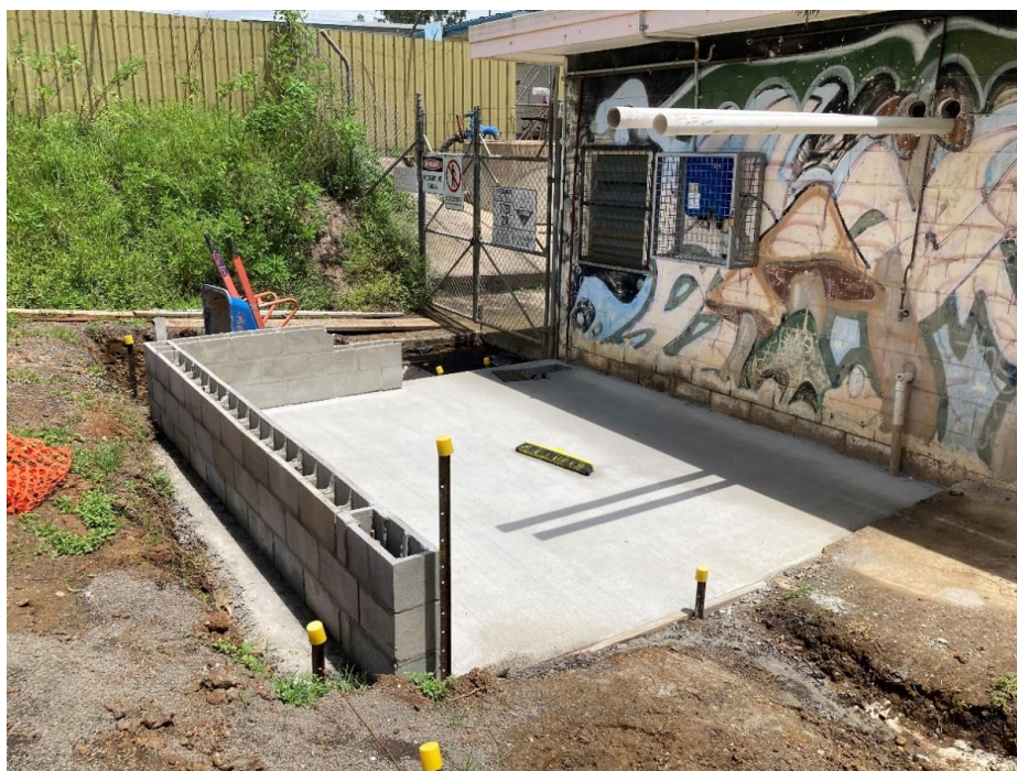
Site preparation for heat pump installation
