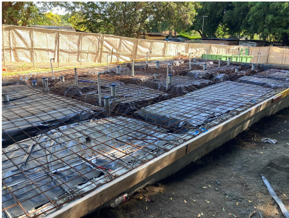
Riverside Caravan Park New Amenities Block Under-slab
