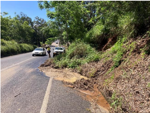
Granite Creek Bridge Approach
