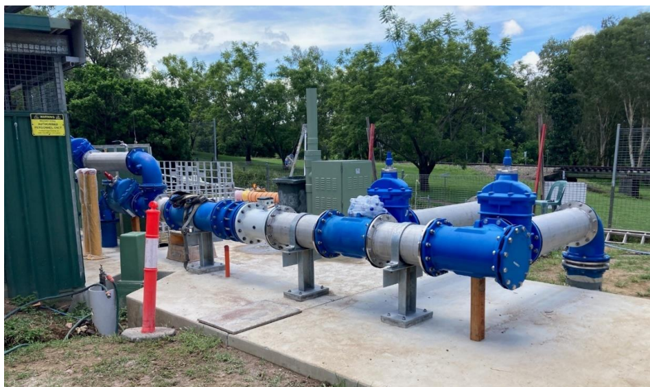
New pump station with external pipe work installation
