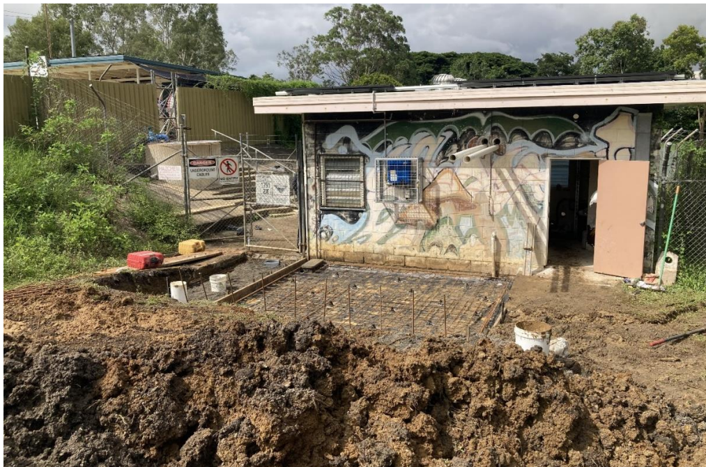
Site preparation for heat pump installation
