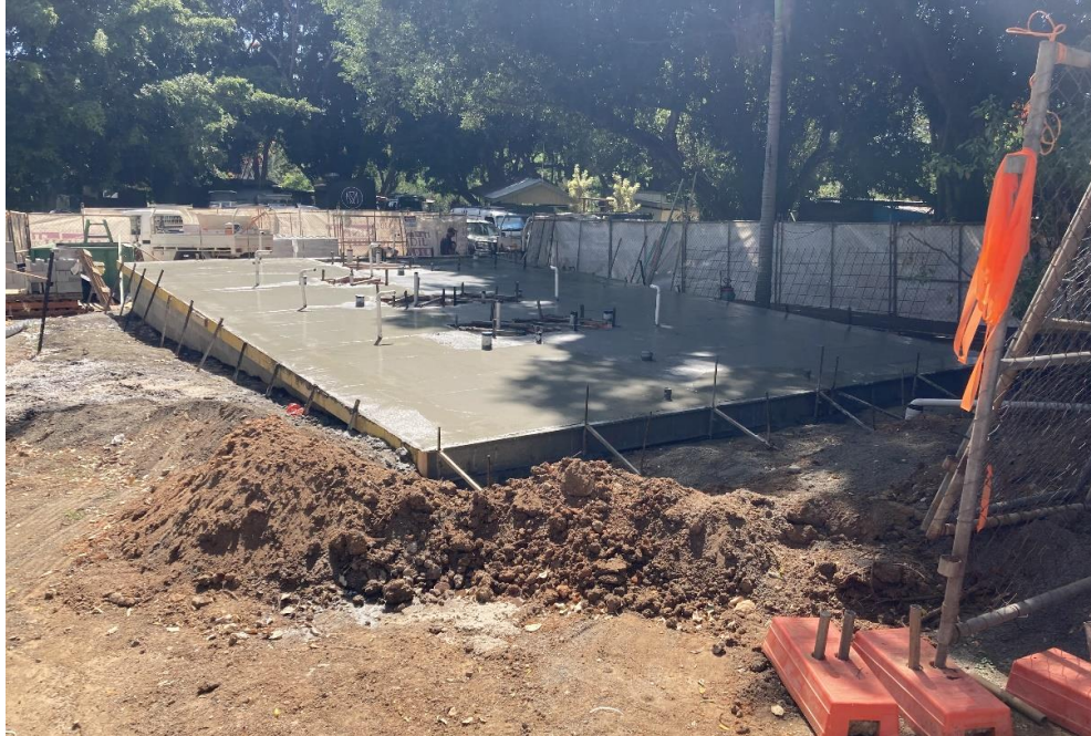
Riverside Caravan Park New Amenities Block Concrete Slab and Plumbing
