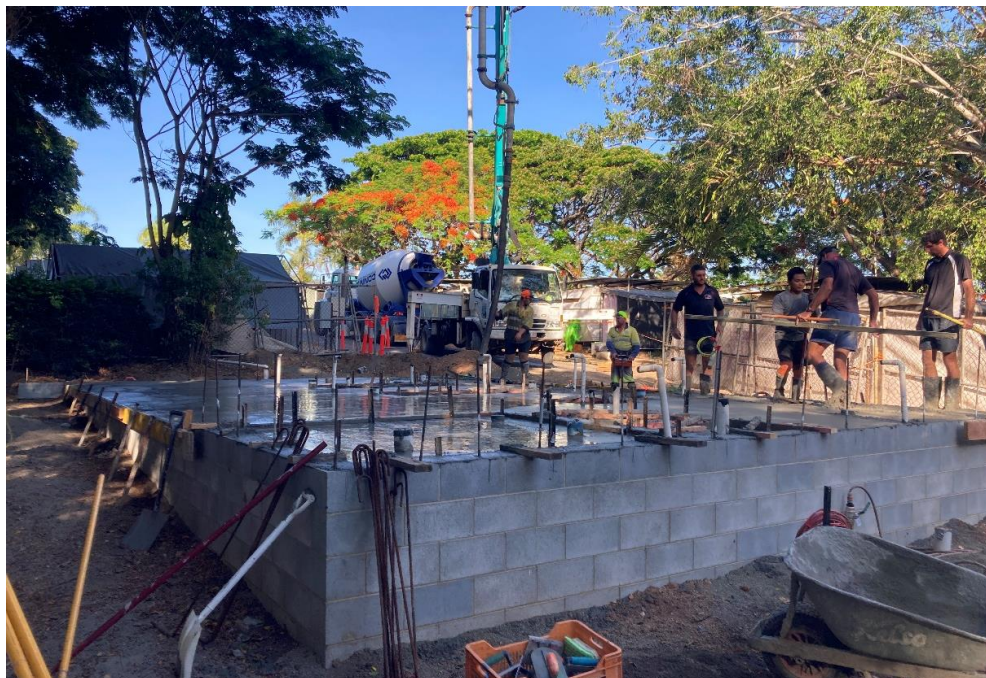
Riverside Caravan Park New Amenities Block Masonry Block Wall Construction
