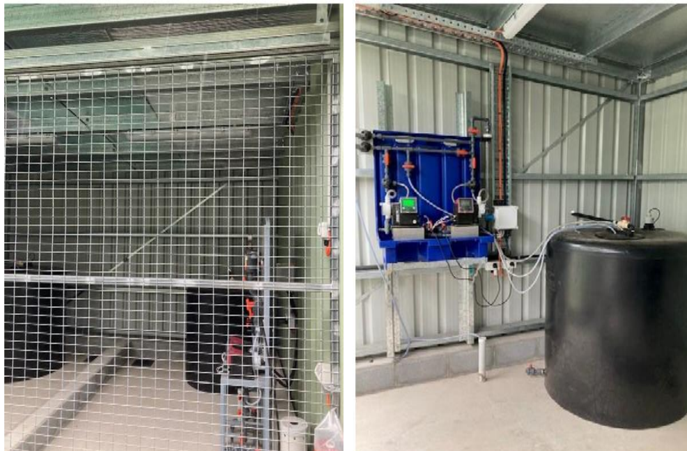
New chemical dosing shed and equipment
