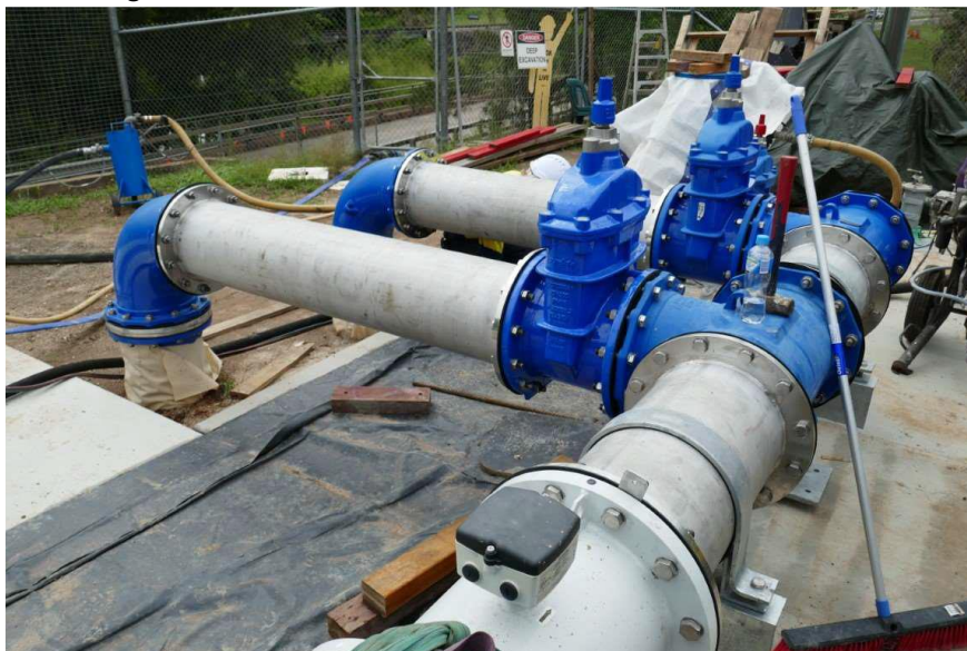
New pump station with external pipe work installation
