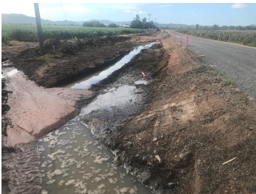
De-watering the site
