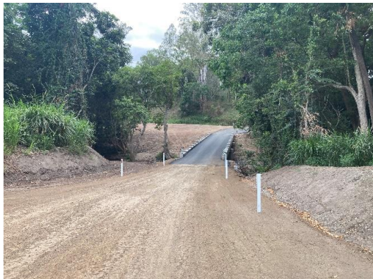
Western bridge approach
