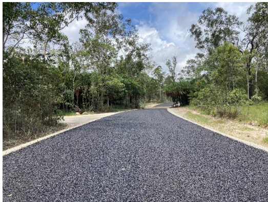
Completed first coat seal - Section B
