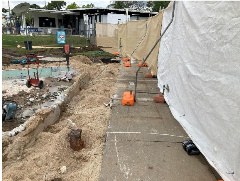
Photo 8 Toddler Pool Decommissioning
