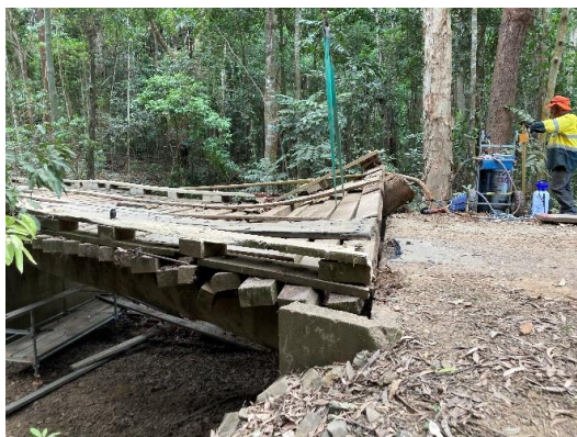
Running plank removal
