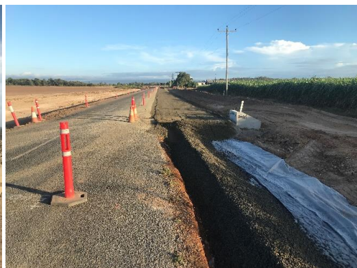
Installation of road base
