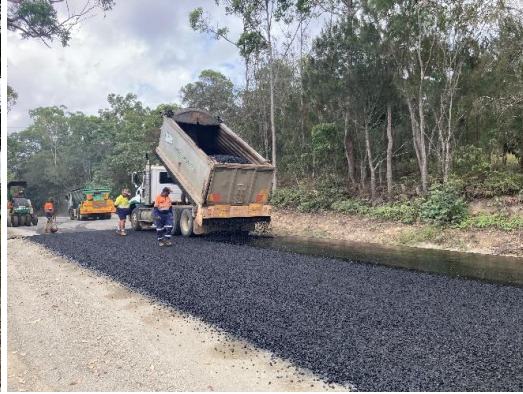
Spreading 16mm aggregate - Section A
