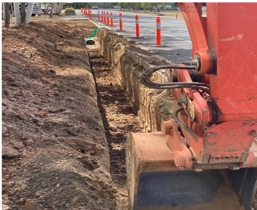
Anzac Avenue installation of the new 300mm diameter PVC Supermain water main
