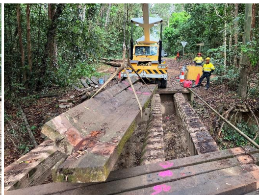
Bridge deck removal
