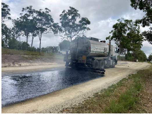
First spray run - Section B
