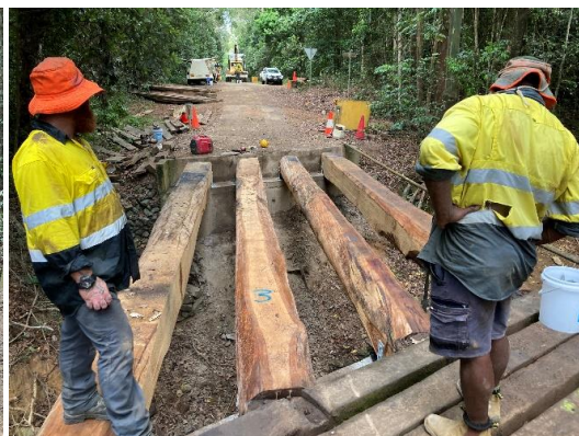
Replaced girders - span one
