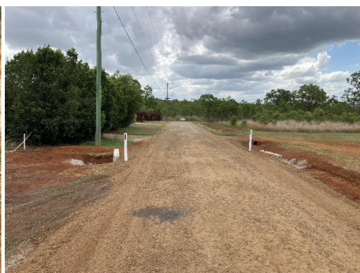
Mclver Road RCBC - complete
