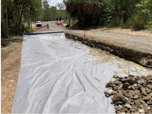
Replacement of unsuitable subgrade - Section B
