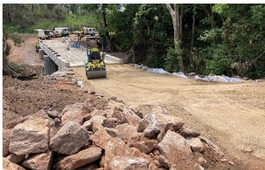
Western bridge approaches
