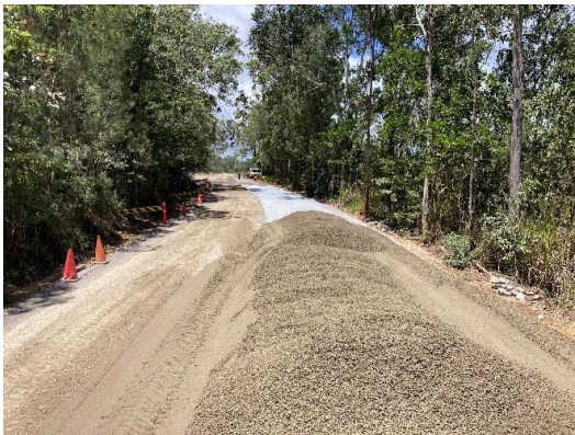
Importing road base - Section B
