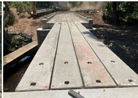
Precast girder installation - western span
