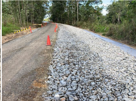
Completed rock mattress - Section B
