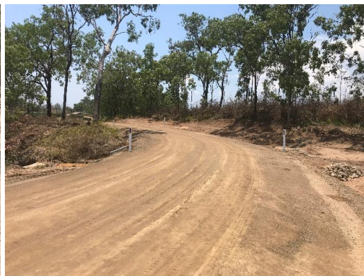
Hawkins Road RCP - completed
