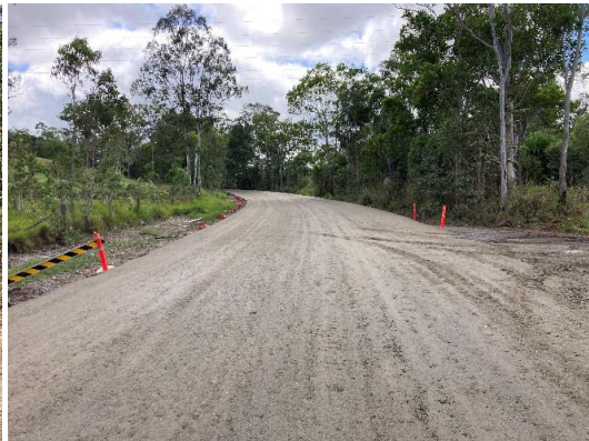
Completed base gravel installation - Section B
