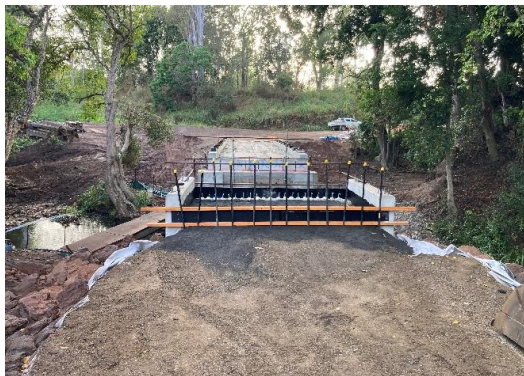
Western relieving slab formwork
