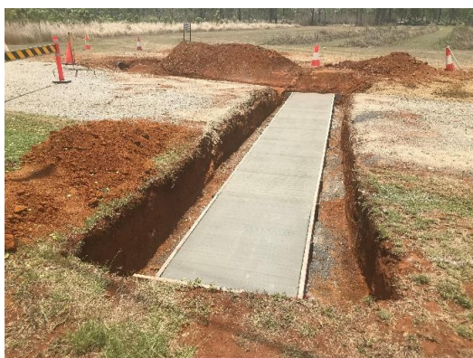
Mclver Road RCBC concrete base
