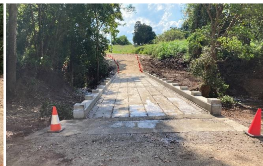
Completed concrete superstructure
