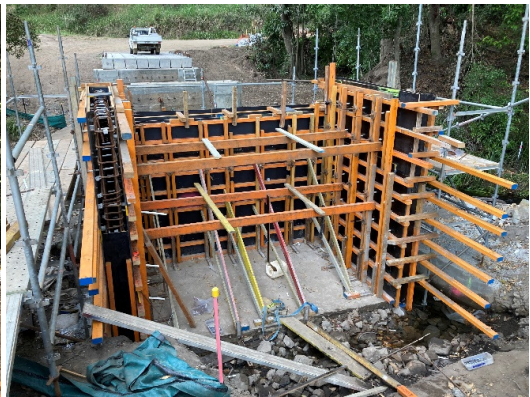
Completed formwork-western abutment
