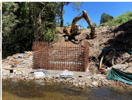
Steel reinforcing in place-western abutment
