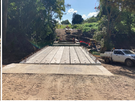
Eastern span girders & kerb units
