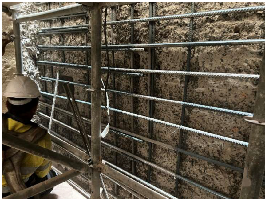
Divider wall remediation Granite Creek SPS
