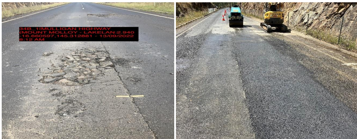
Mulligan Highway Pavement Repairs
