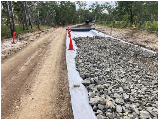
Back filling with crushed rock
