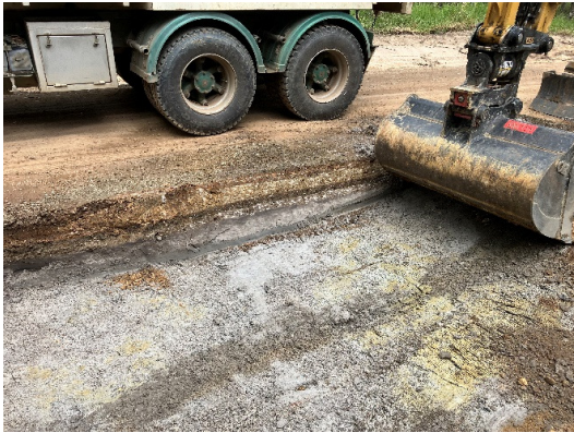
Removal of unsuitable subgrade
