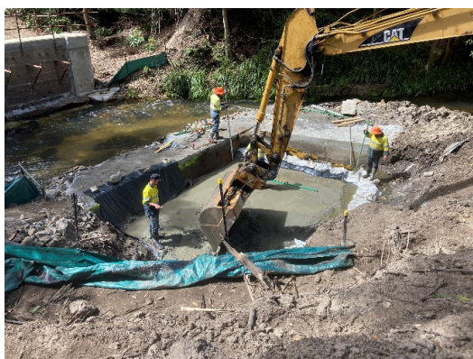
Pouring concrete blinding layer- western abutment
