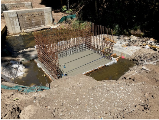
Concrete base-western abutment
