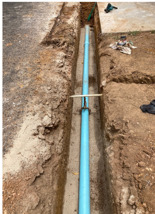
Molloy Street installation of the new 150mm diameter PVC Supermain
