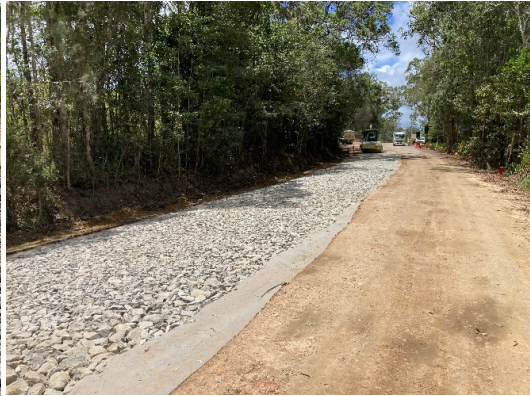
Completed subgrade replacement section
