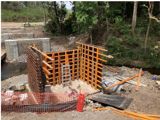
Commencing formwork-western abutment
