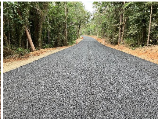
Section C - Completed Two Coat Seal
