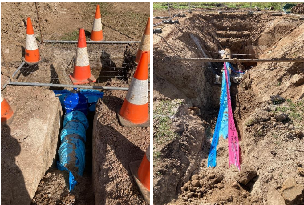
Installations of the new 300mm diameter PVC Supermain along Moody Street
