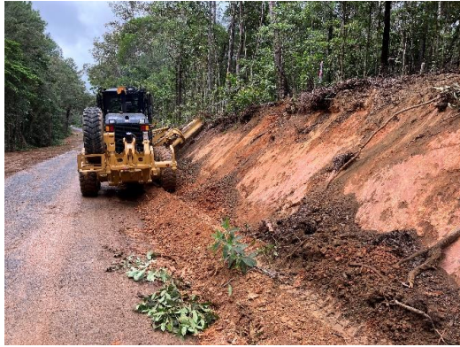
Section C - Earthworks
