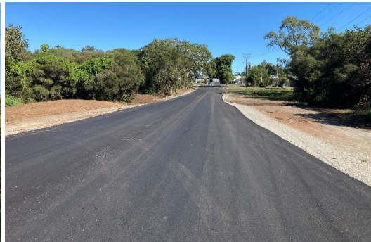
Reynolds Street (after)
