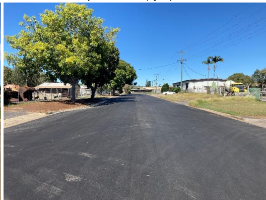
Reynolds Street (after)
