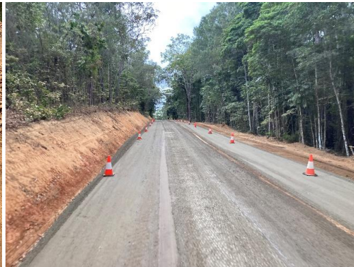
Section C - Completed Base Layer Widening
