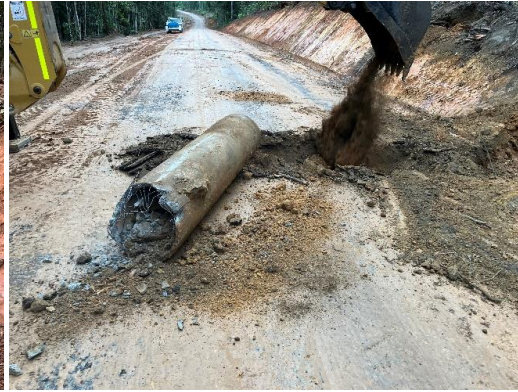
Section C - RCP Removal
