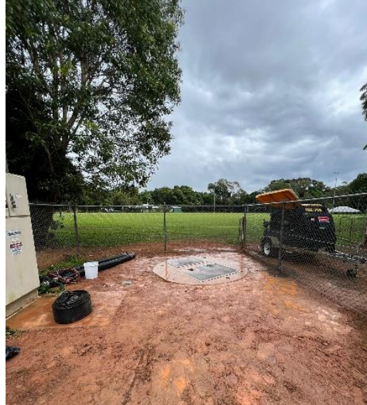
Works completed at Arara Street, Kuranda
