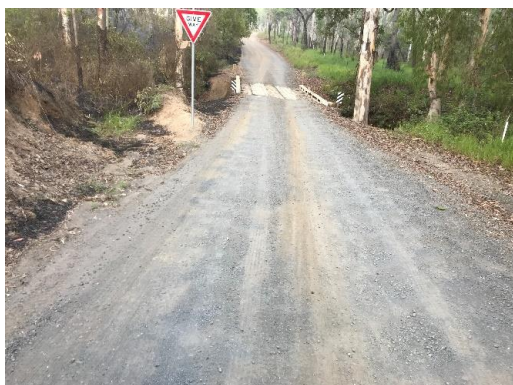
Davies Creek Road bridge (before)
