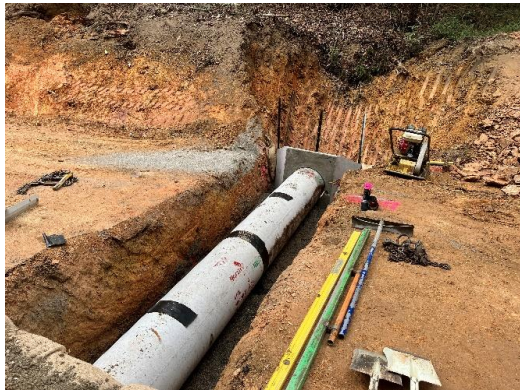
Section C - RCP Replacement
