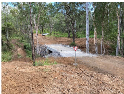
Davies Creek Road bridge (after)
