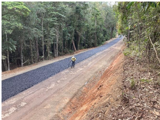
Section C - First Coat Bitumen Seal 16mm
