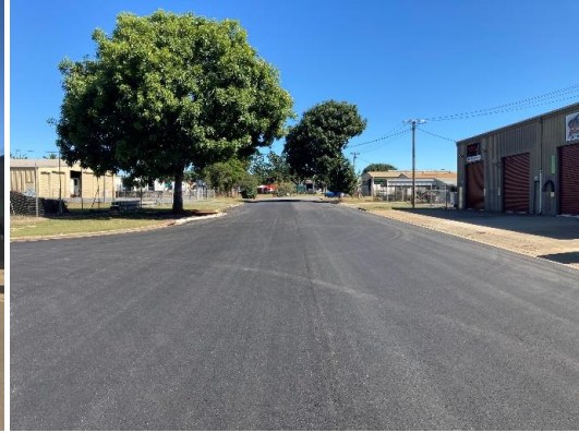
Reynolds Street (after)
