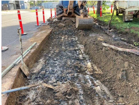
Removal of failed pavement & damaged K&C
