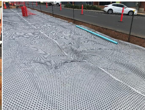
Geofabric covering replaced unsuitable material
