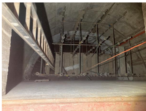
Internal pump station stripped out
