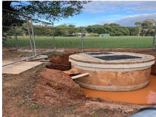
Site excavated to install root barrier
