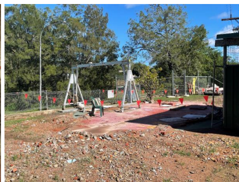
Demolition of the upper pump station structures
