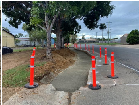
Site ready for new K&C installation
