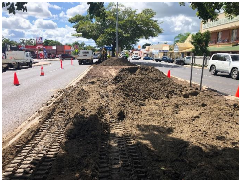
Preparation of new northern median garden bed
