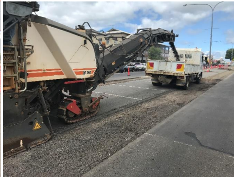
Milling existing seal from centre car parks
