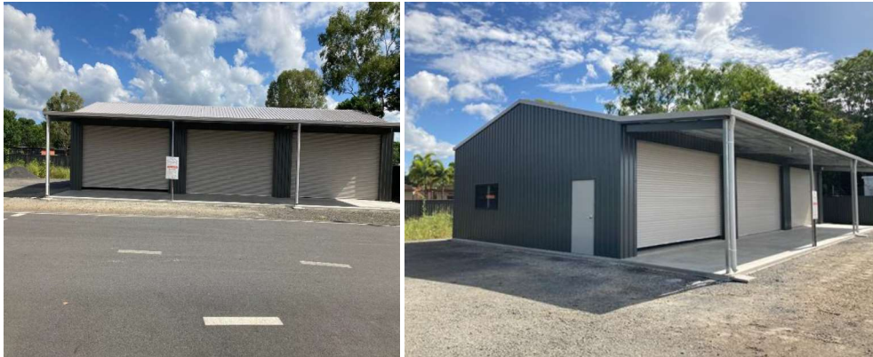
Newly constructed Buy Back Shop Shed
