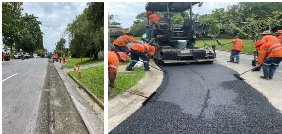
Road reinstatement over the water main installation
