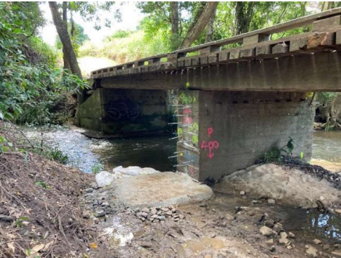
Pier dowels installed
