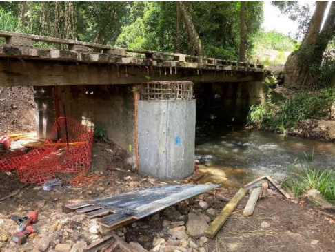
Completed Pier Extension
