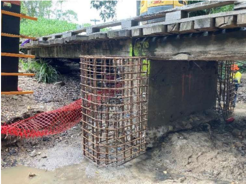
Pier reinforcement in place
