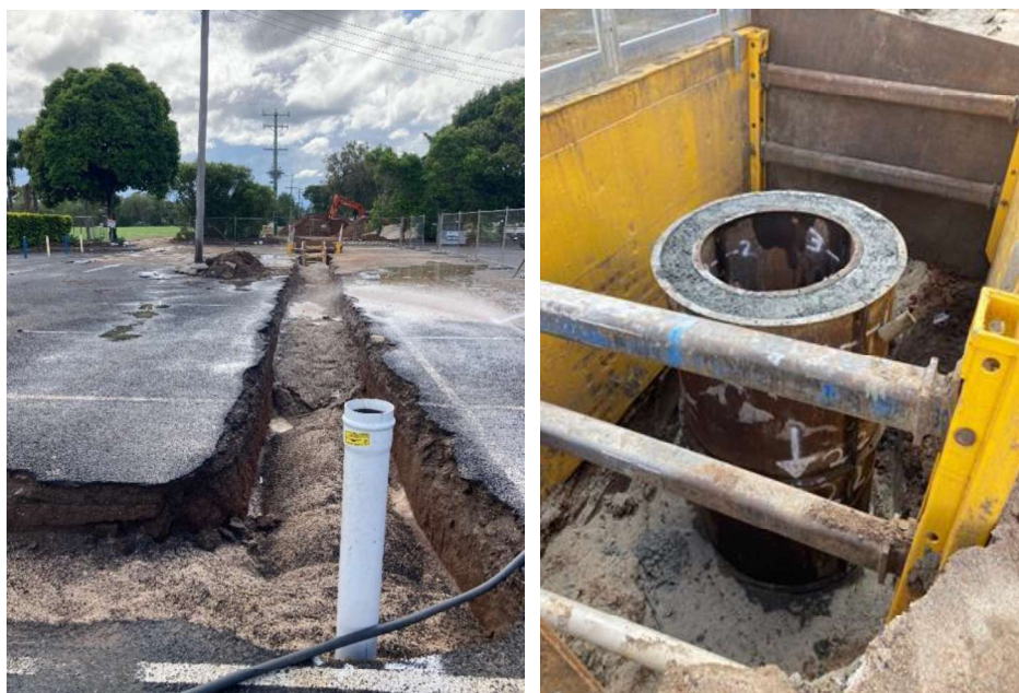
Installations of the new gravity sewer main and manholes
