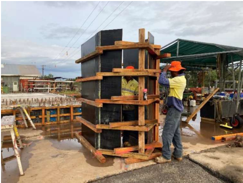
Preparing formwork for pier extension
