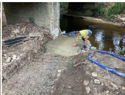
Completed pier extension footing
