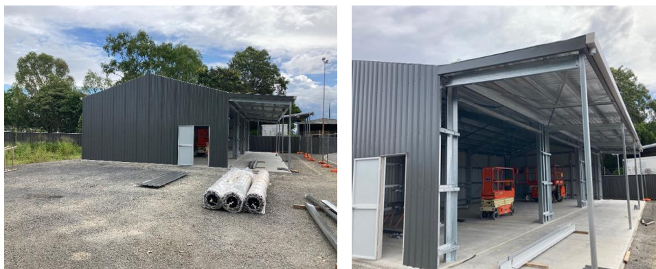
New Buy Back Shop Shed under construction
