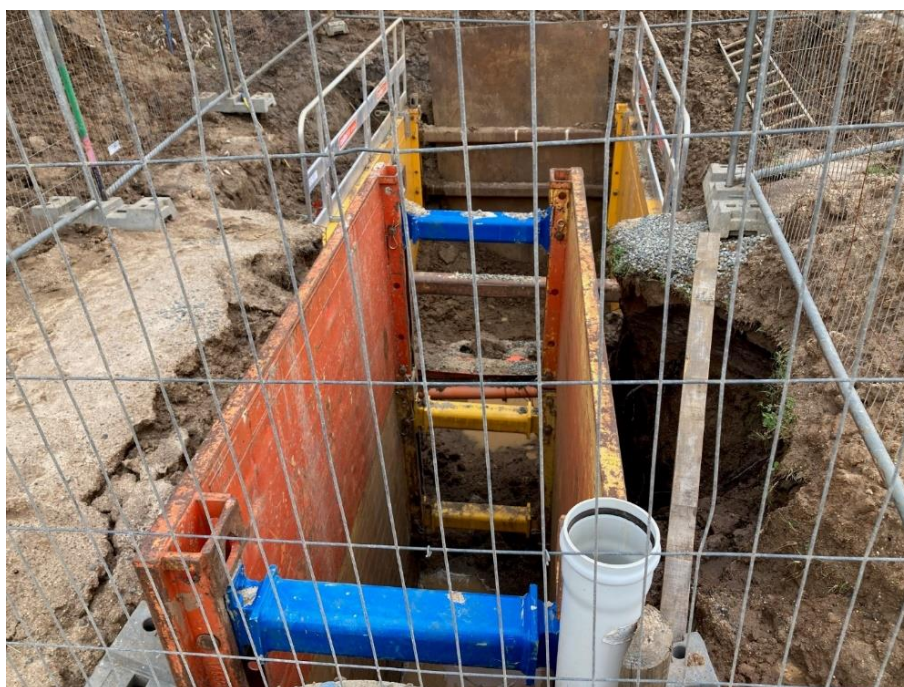
Excavation works for gravity sewer main
