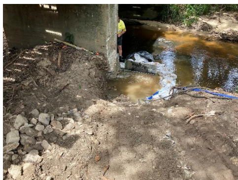
Preparing for pier extension footing
