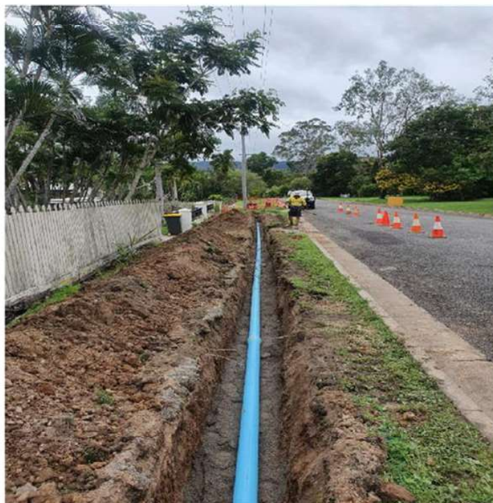
Installation of new water main on Fraser Rd Mt Molloy
