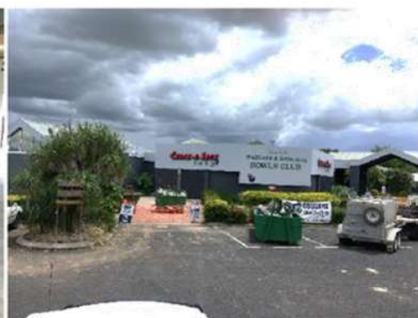
View of demolished area to be purposed for the new Library
