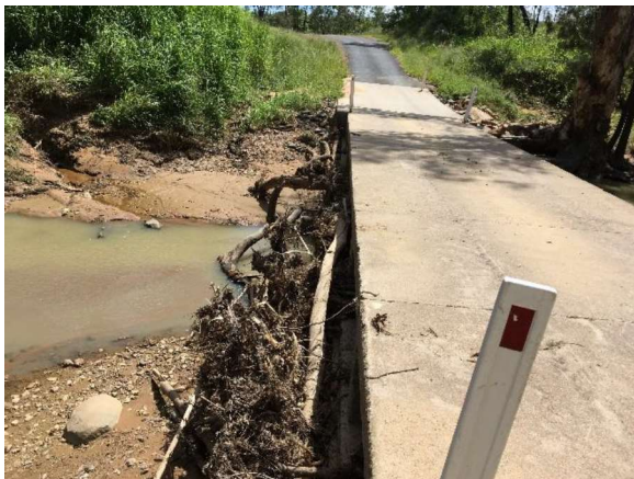
Leadingham Creek Road Causeway
