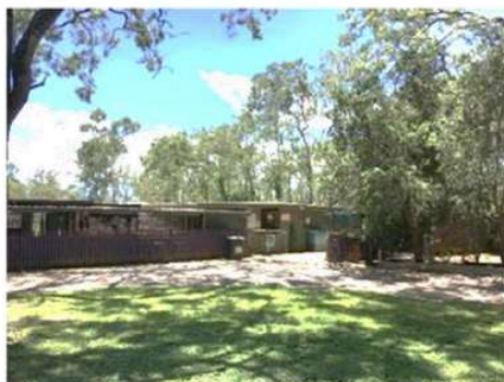
Existing Pound facility
