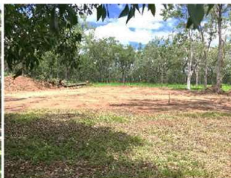
Cleared site for new pound facility
