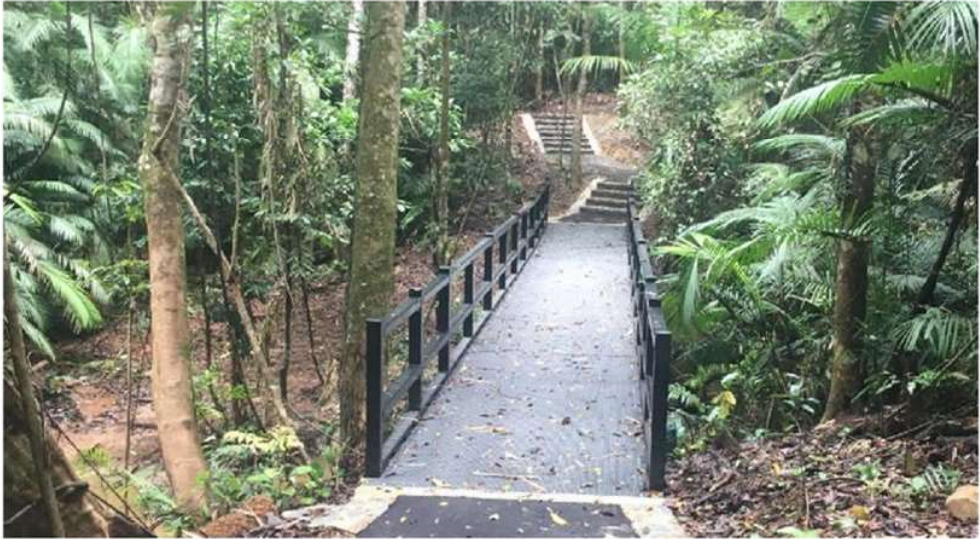
Bridge 7 Platypus Creek National Park Section
