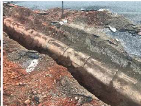
Failing Existing Stormwater System
