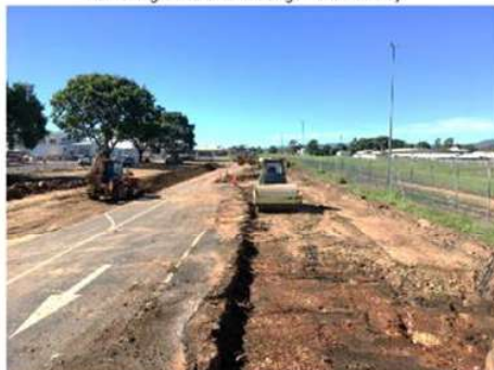
Compacting Select Fill
