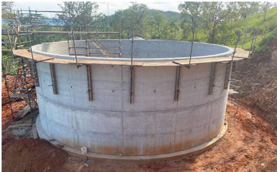
Formwork removed follow curing of concrete
