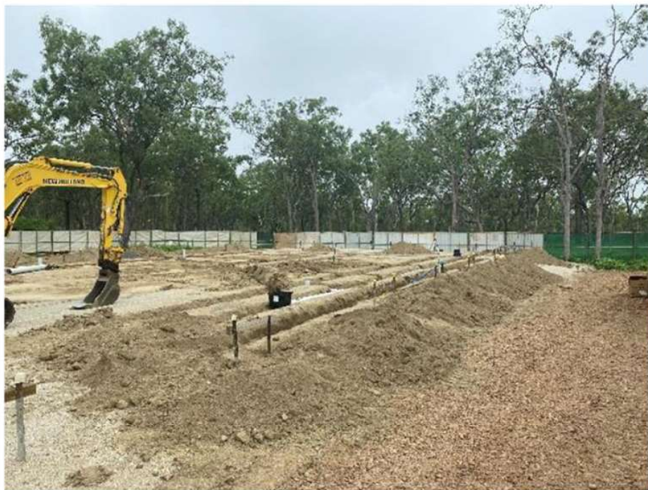
Building Pad partially prepared for substructure
