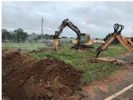
Removing Slabs and Footings - Old Railway
