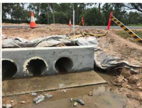
Completed Apron and Headwall
