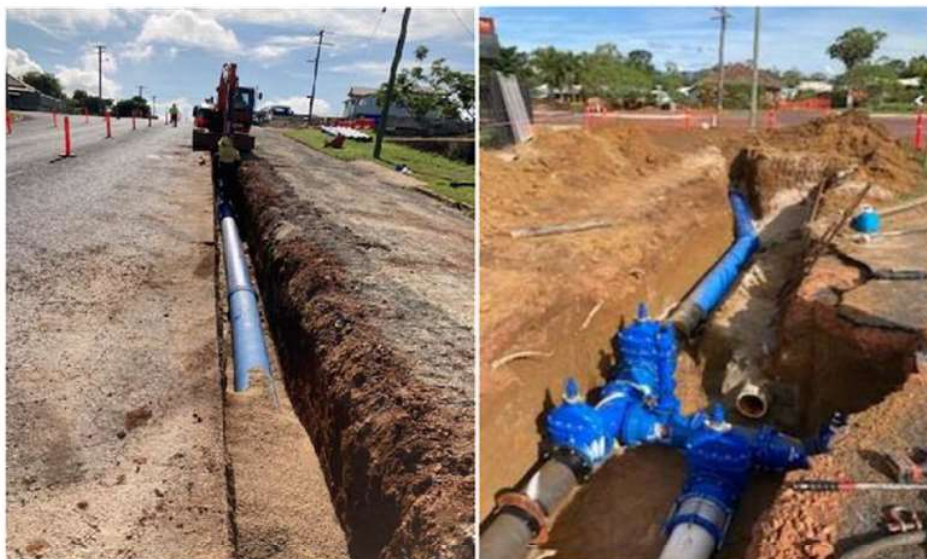
Construction and installation of the new 300mm ductile iron water main and cut-in and valve arrangement at the Rankin Street and Chewko Road intersection.
