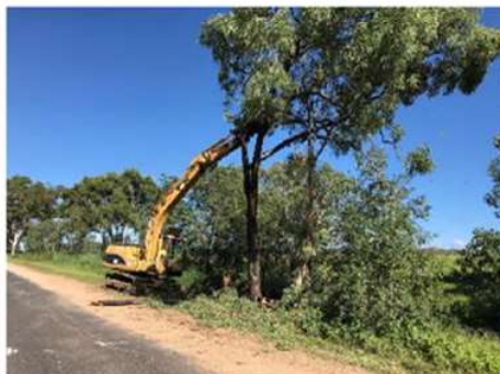
Clearing and Grubbing
