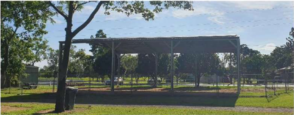
Centenary Park - Completed solar structure and panels
