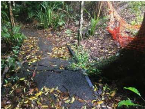
Jungle Trail Ch.60 - Raised Damaged Section
