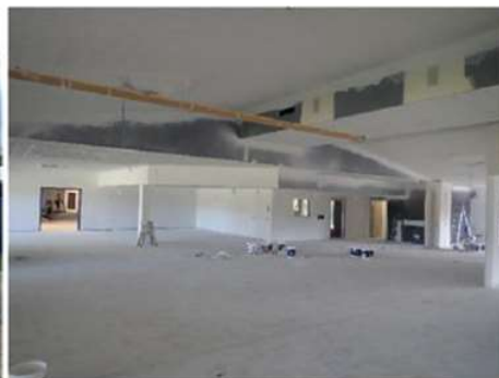
Partial internal paint
