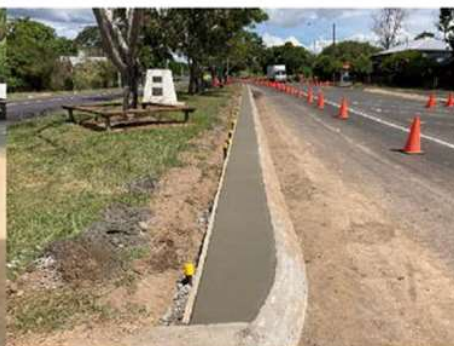
Completed Maintenance Kerb
