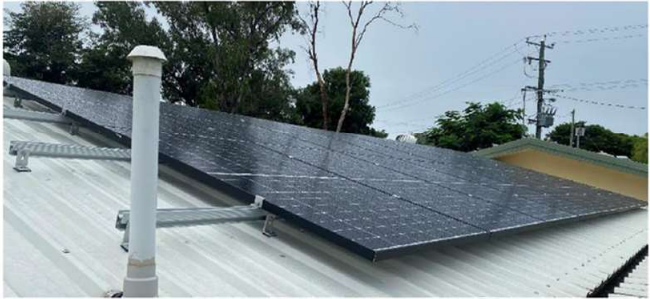
Mareeba Swimming Pool - Completed installation on Swimming Club Roof
