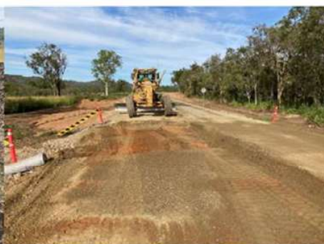
Base Layer Installation
