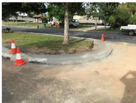
Completed Replacement of failed Kerb
