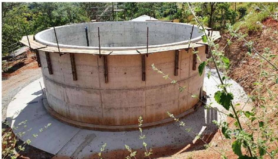
New Concrete Path around Reservoir
