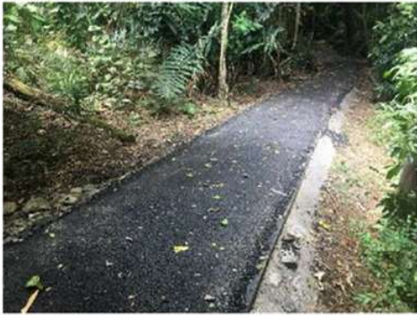
Jungle Trail - Refurbished edge stanchion & asphalt overlay
