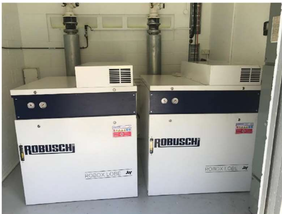
Newly installed rotary lobe blowers
