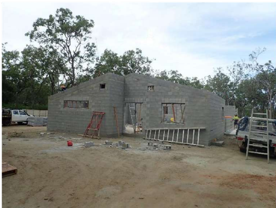
Blockwork nearing completion
