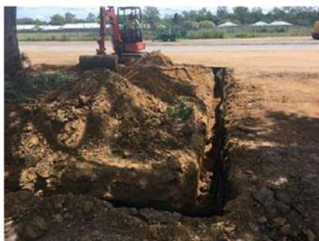
Root Guard Installation
