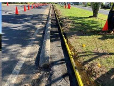
Preparation for Maintenance Kerb
