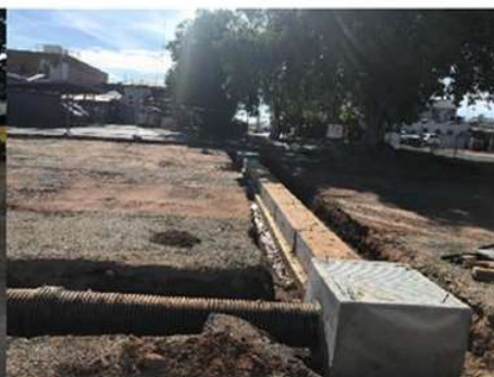
Stormwater System Installation
