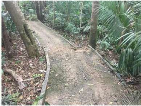
Jungle Trail - Section with old concrete steps removed
