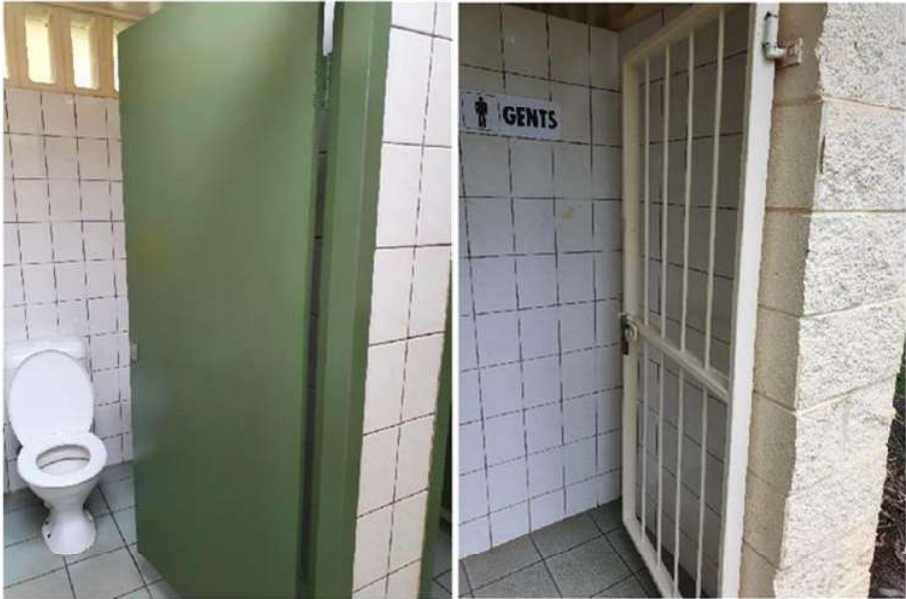
Centenary Park Completed Internal Works
