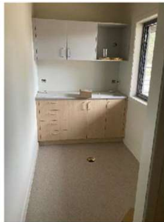
Internal kitchen fit-out with vinyl sheet flooring
