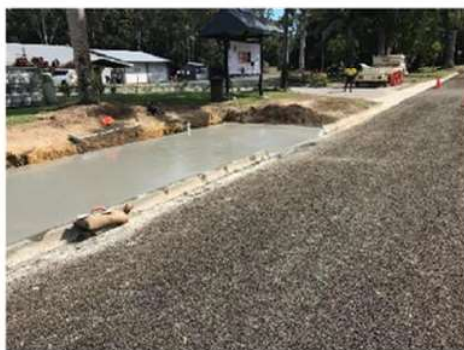
Bus shelter slab
