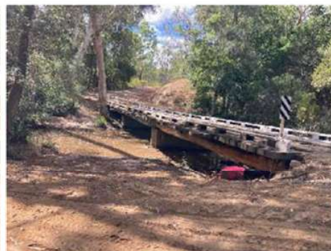
Completed bridge works
