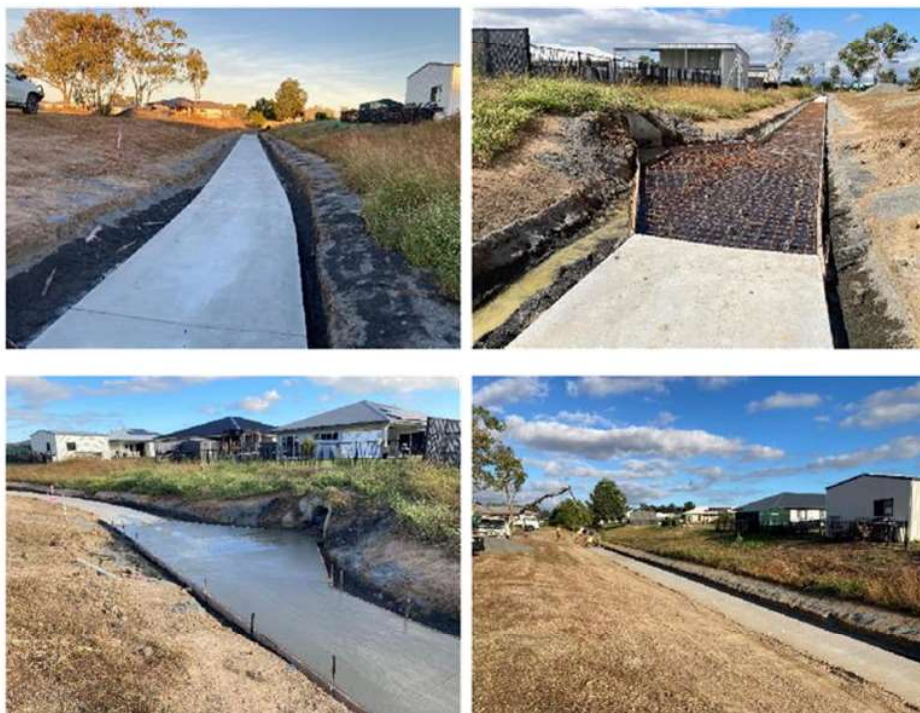
Construction of concrete invert
