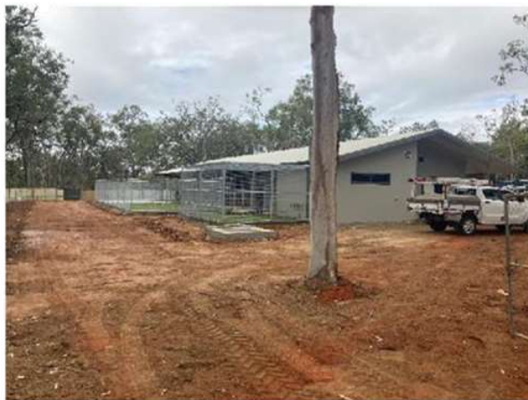
External works to the northern side including cat and dog runs
