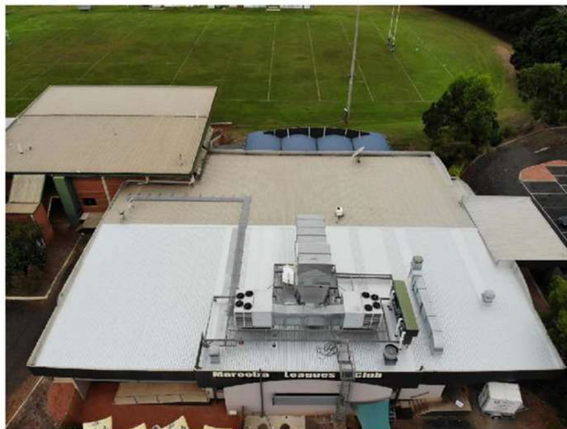
Completed works seen from a drone perspective
