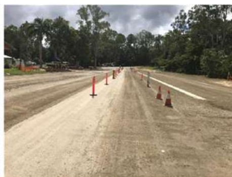
Completed unsealed pavement
