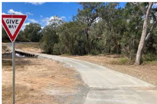
South western end of culvert (after)
