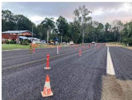
Completed sealed pavement
