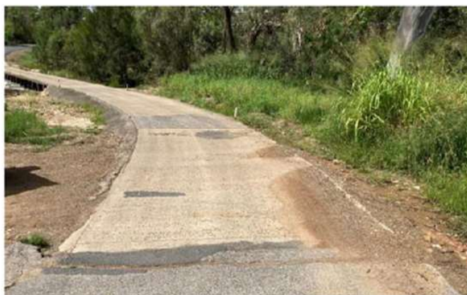
South western end of culvert (before)
