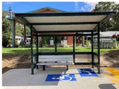
Completed bus shelter
