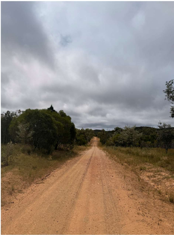
East View Hales Siding Road entry to Mullock Heap 1
