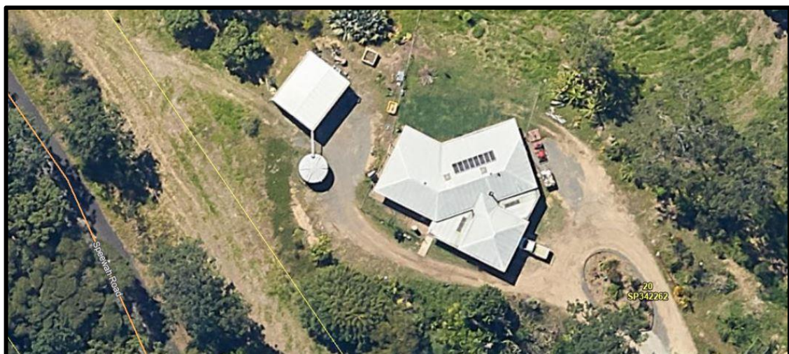
Figure 1: Existing Dwelling House on Speewah Rd frontage (Qld. Globe).
