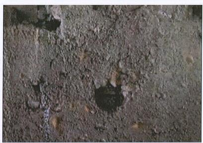
Photograph 6 - Concrete condition, including exposed reinforcement
