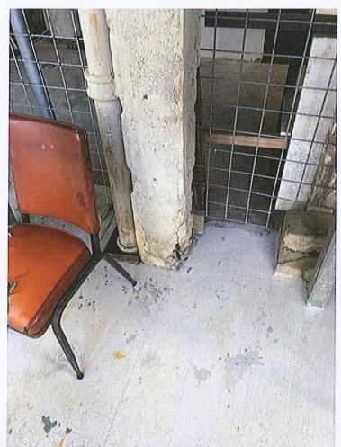
Photograph 13 – Concrete column with spalled concrete and exposed reinforcement
