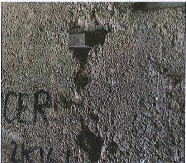
Photograph 9 - Concrete condition and timber block from construction, typically used to support reinforcement
