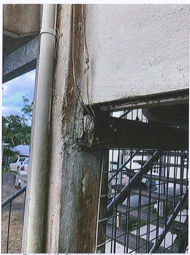
Photograph 12 - Displaced and unsupported timber bearer
