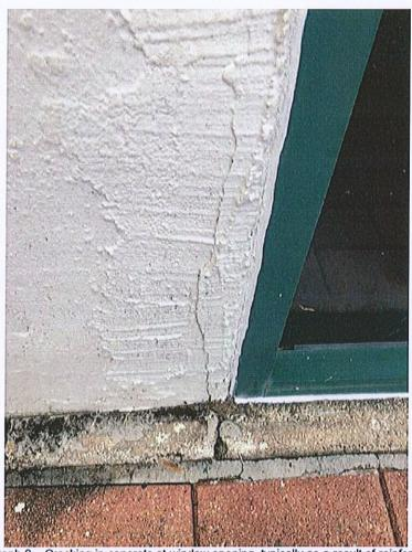
Photograph 3 – Cracking in concrete at window opening, typically as a result of reinforcement expansion due to exposure and rusting
