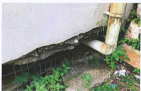
Photograph 1 - Spalled concrete on concrete beam of north eastern corner of structure
