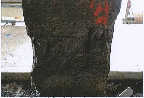
Photograph 2 - Exposed reinforcement on concrete column
