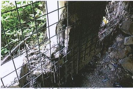
Photograph 5 - Deteriorating concrete column
