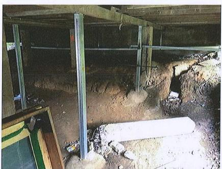
Photograph 10 - Multiple existing interior columns replaced with new steel columns
