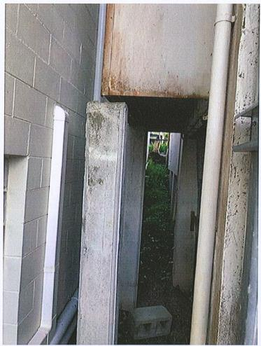
Photograph 14 - Column not supporting floor framing above (gap between column and floor framing)
