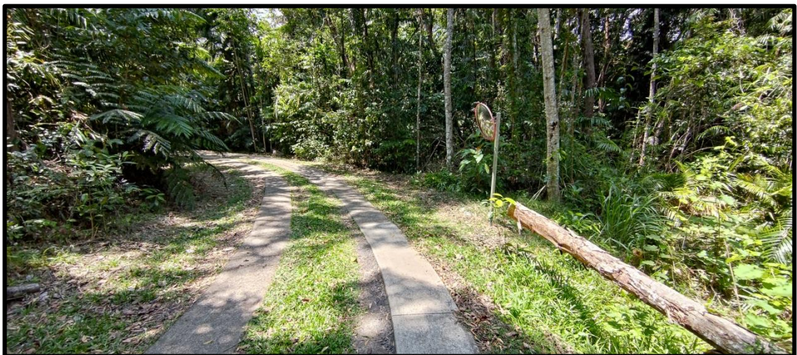
Figure 3: Existing on-site concrete driveway treatment (STP).
