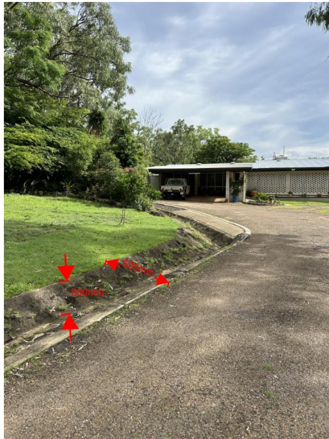
Figure 8: Existing Stormwater Drainage Concrete/Rock Channel
