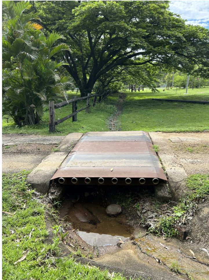
Figure 10: Existing Open Rock lined Channel.
