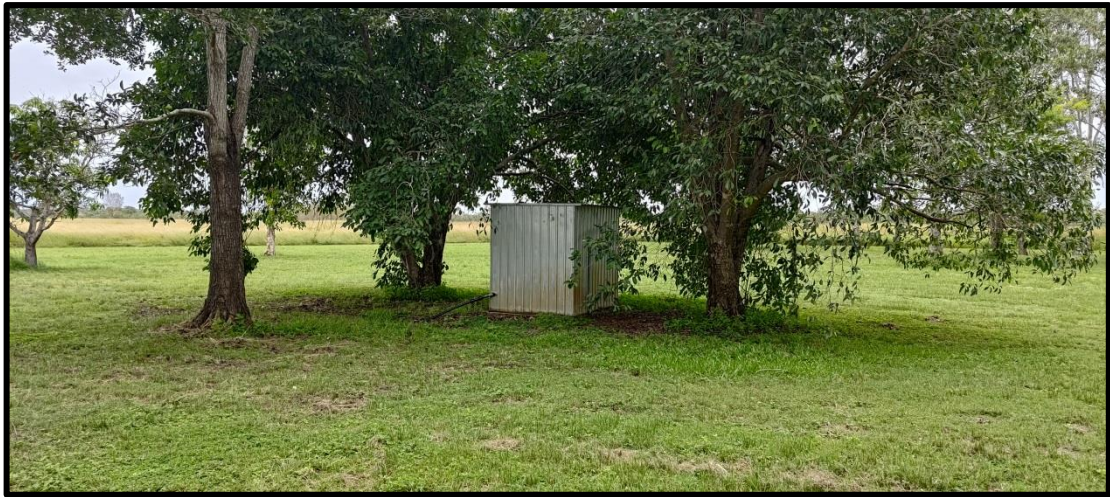
Figure 10: On-site bore water supply (STP).
