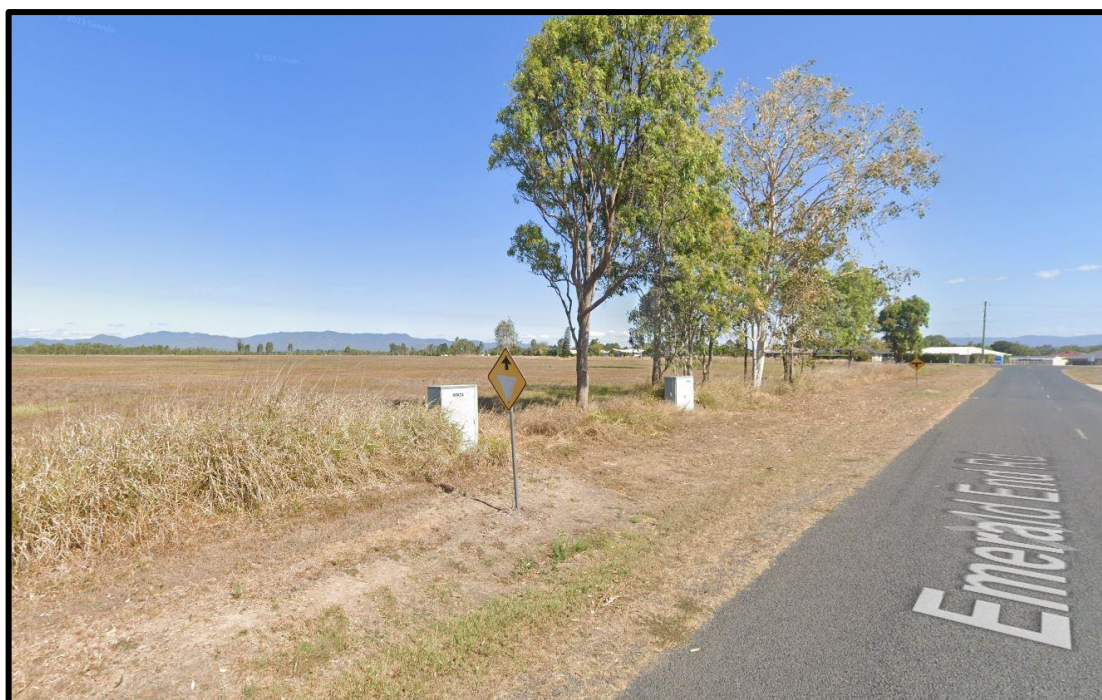
Figure 9: Reticulated electrical provisions on Emerald End Road (Google Maps).
