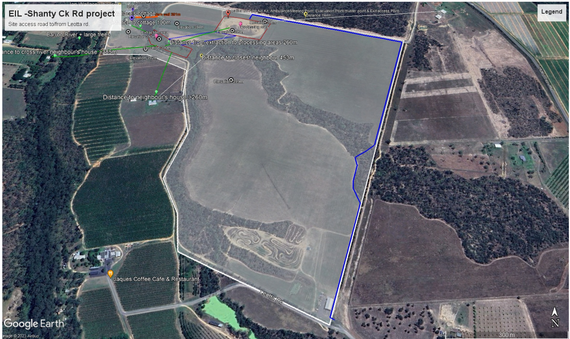
Figure 2b – site access road
