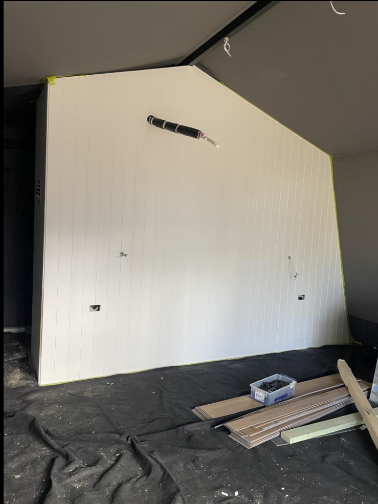
Separates bathroom and bedroom
