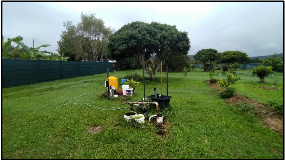
Figure 12: Bore water supply for existing Dwelling (near Dwelling House).
