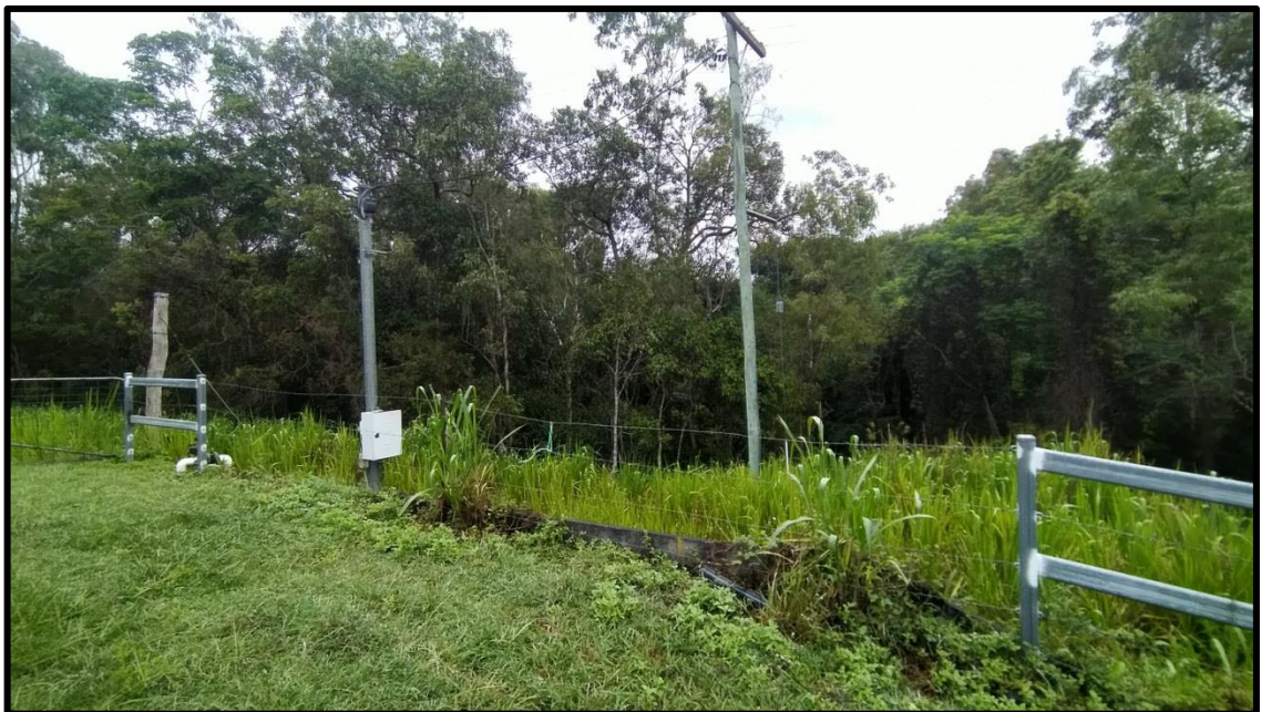
Figure 10: Reticulated electrical provisions site photo [tile 10].
