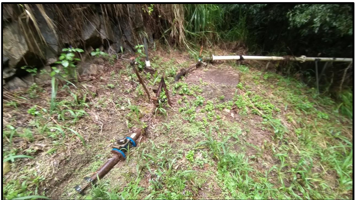
Figure 13: Clohesy River water supply pump site provisions (rear of site).
