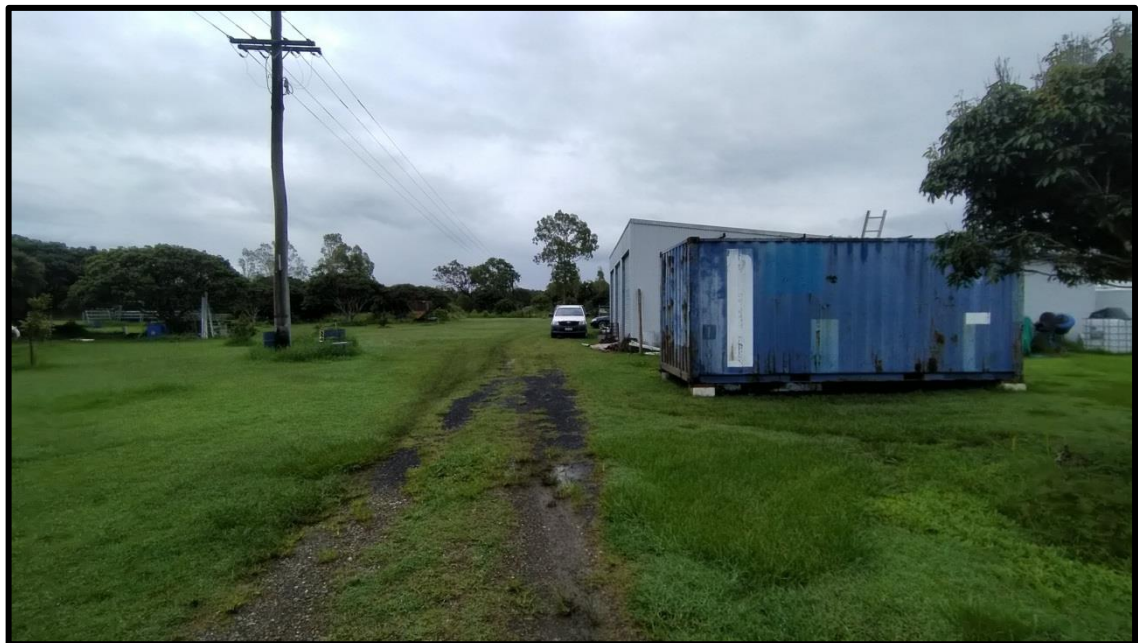
Figure 8: Reticulated electrical provisions site photo [tile 5].
