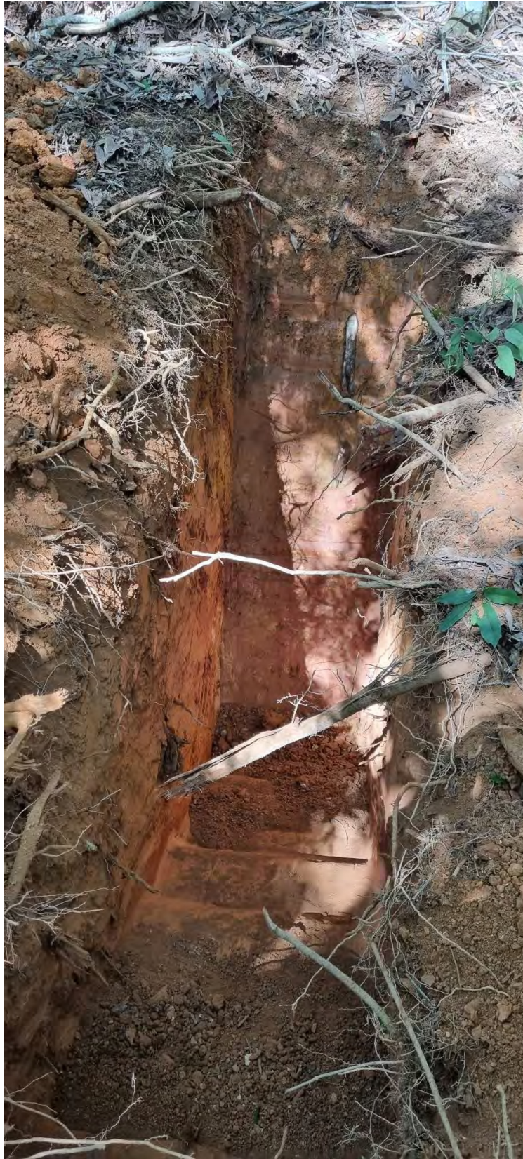
PHOTOGRAPH 5: Test Pit 4 on Lot 21
