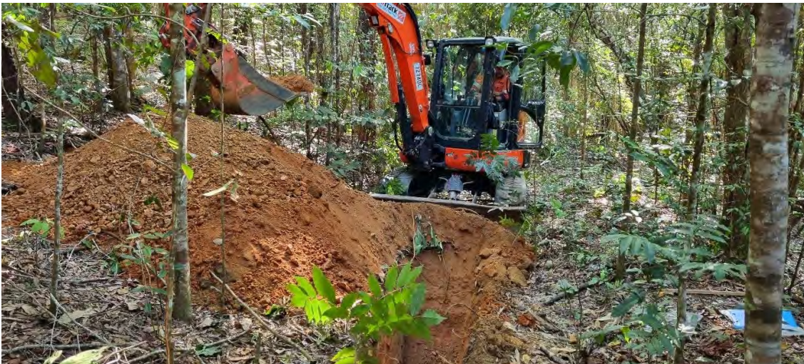
PHOTOGRAPH 16: Spoil from Test Pit 2 on Lot 24
