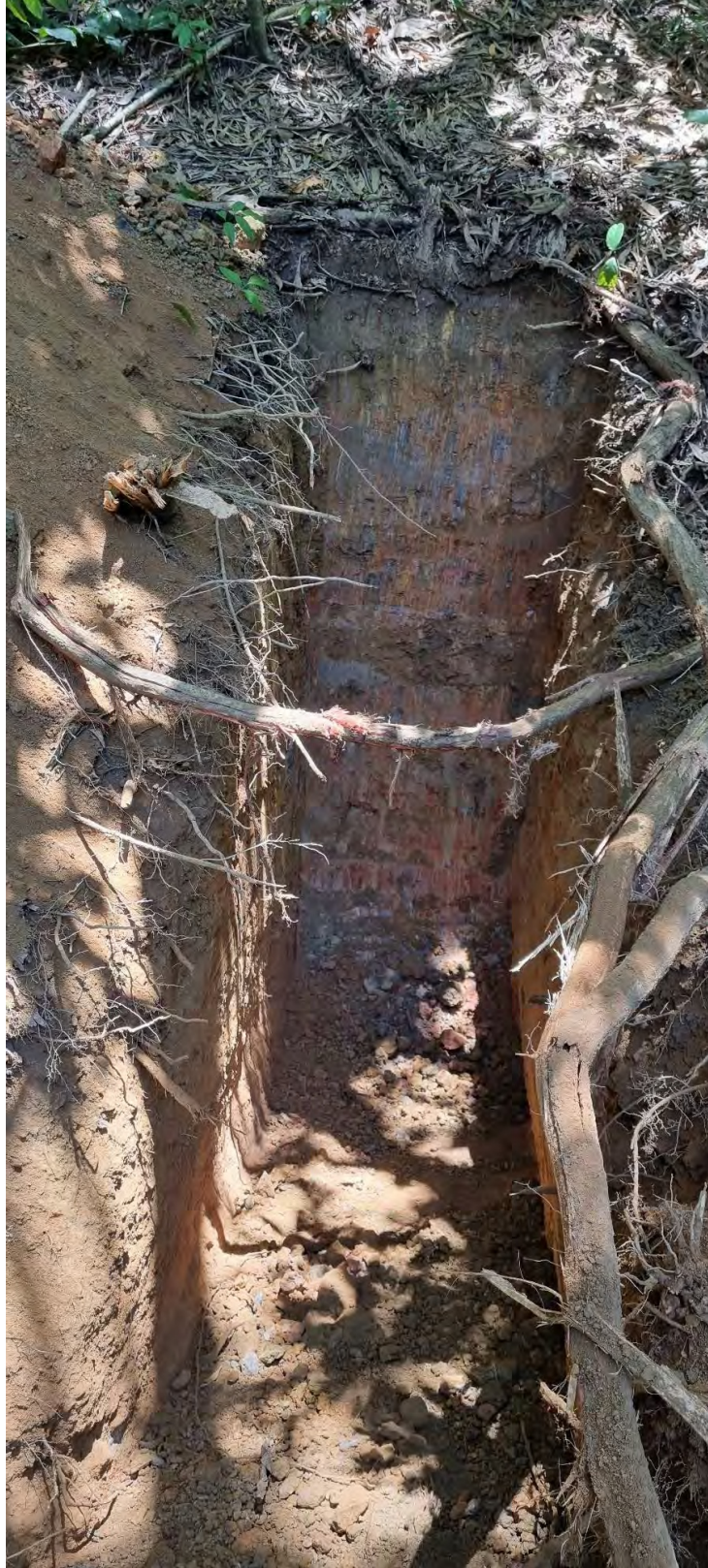
PHOTOGRAPH 2: Test Pit 7 on Lot 20
