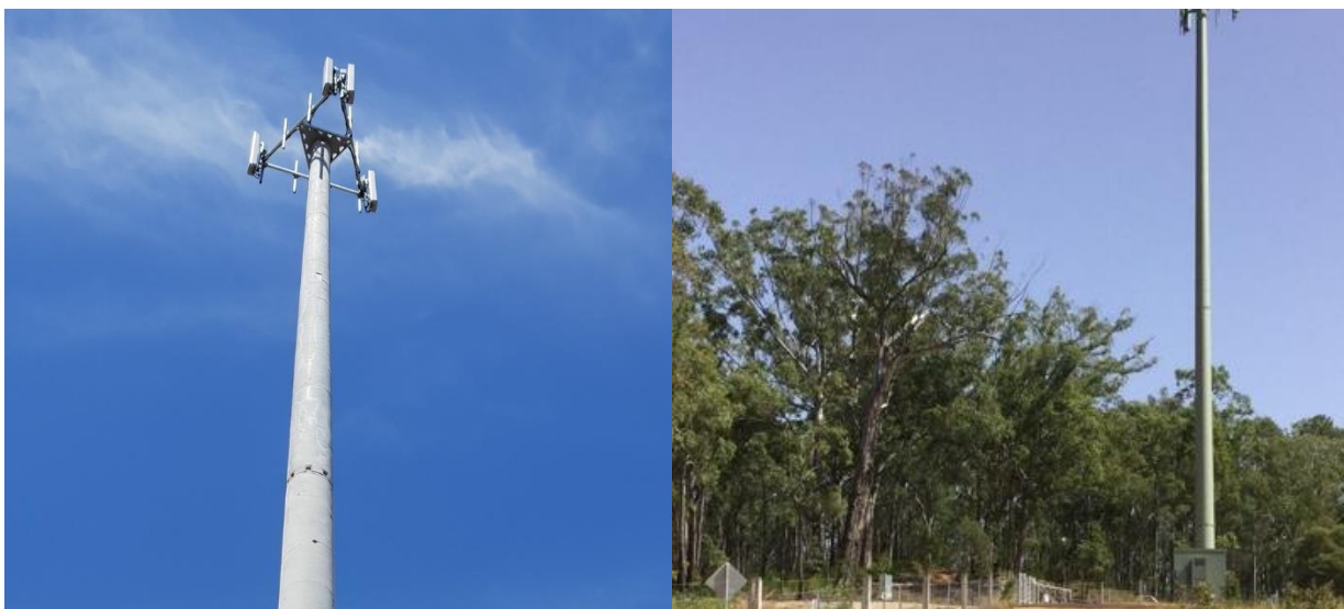
Figure 19: (Left) As constructed example of low reflectivity of concrete monopole against sky backdrop. (Right) As constructed example of colour-treated concrete pole against vegetated and sky backdrop (Source: Ventia 2022)
