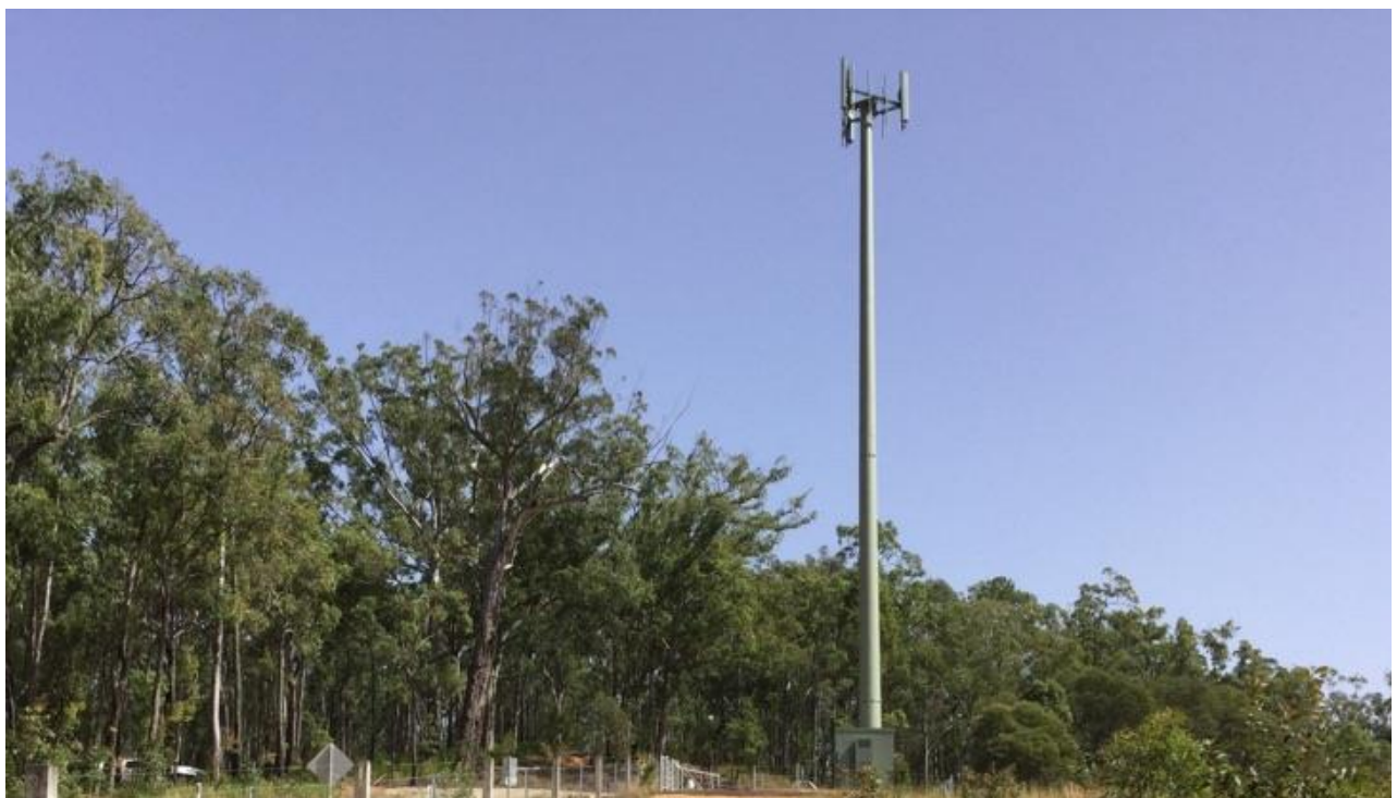
Figure 9: Image of example 40m monopole with headframe and antennas all colour-treated mist-green. Note that image does not include solid coloured fencing surrounding compound (Source: Ventia, 2020)
