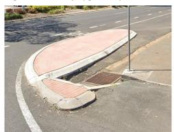
Figure 29 Kerb Inlet Pit on Western Side of Byrnes Street at the Byrnes Street/Jacobsen Street Intersection (Google Street View, Approximately 1km downstream from site)
