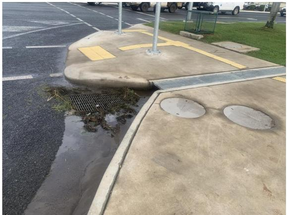
Figure 21 Grated Inlet Pit at Byrnes Street/Rankin Street Intersection – 1 (Note: Further Restriction of Channel Flow Created by the Grated Drain as Part of the Intersection Upgrades. The Grated Inlet Pit was Blocked by Debris and was Cleared During Inspection.)
