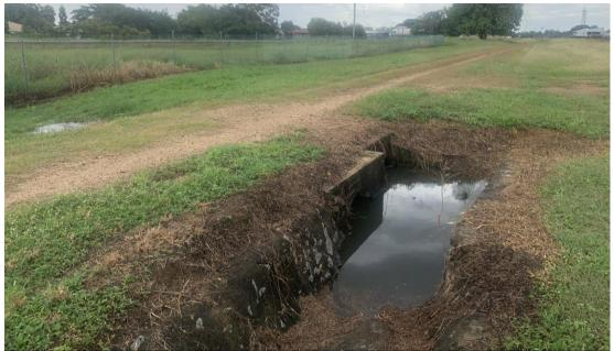
Figure 23 Culvert Crossing (1×900mm RCP and 1×1200mm×600mm RCBC) under Abandoned Railway Formation – 1 (Southwest from the Site, the Tree is on Western Site Boundary)
