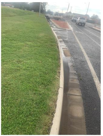
Figure 20 Kerb and Channel on Rankin Street – 2 (Looking West Near the North-eastern Corner of the Site, Note the High Point at the Railway Line Represents the Catchment Boundary to the West)
