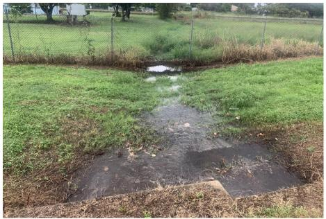
Figure 25 Table Drain West from the Abandoned Railway Formation (Looking West Downstream, Showing the Culvert Crossing Under the Operating Railway)
