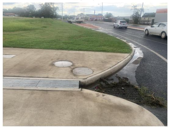
Figure 22 Grated Inlet Pit at Byrnes Street/Rankin Street Intersection - 2
