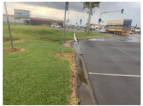
Figure 18 Kerb and Channel on Byrnes Street - 2 (Note: Restriction in Flow Path Capacity Created by the Traffic Island)
