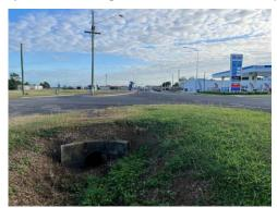
Figure 28 Table Drain and Headwall on Western Side of Byrnes Street at the Byrnes Street/Herberton Street Intersection (Looking North. Note: Surface Flows not Captured at This Point Will Bypass the Southern Pipe System and Travel North along the Site Road Frontage to the Recently Upgraded Byrnes Street/Rankin Street Intersection)
