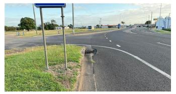
Figure 27 Kerb Inlet Pit on Western Side of Byrnes Street at the Byrnes Street/Herberton Street Intersection (Looking North. Pipes cross from right to left in direction of flows)
