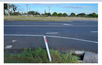
Figure 26 Kerb Inlet Pit on Eastern Side of Byrnes Street at the Byrnes Street/Herberton Street Intersection (Looking West downstream)
