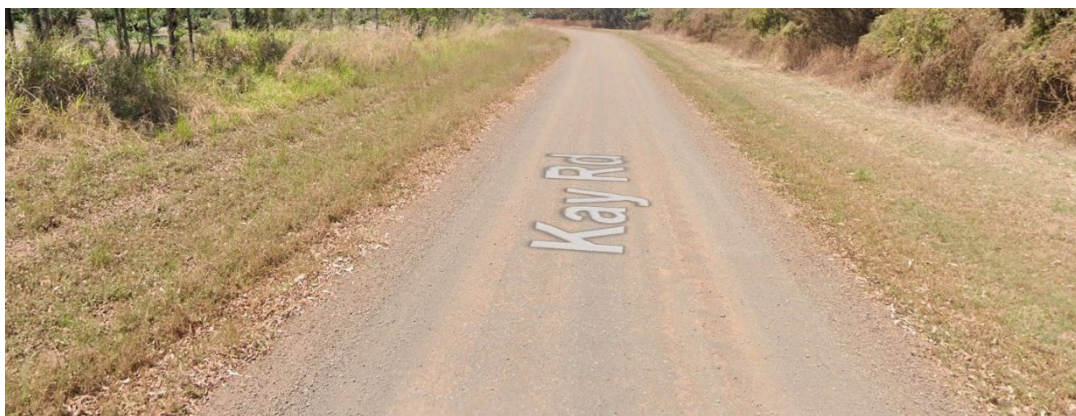
Photograph 2.27 – Kay Road Chainage 3900
