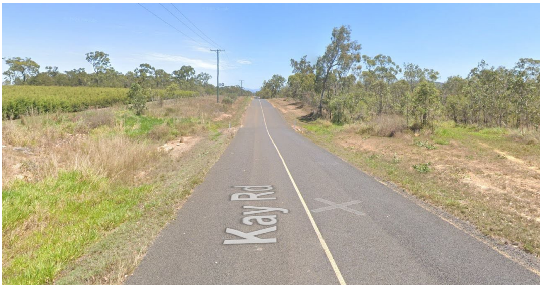
Photograph 2.18 – Kay Road Chainage 550
