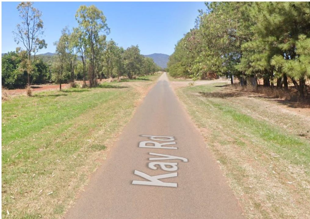
Photograph 2.24 – Kay Road Chainage 2550
