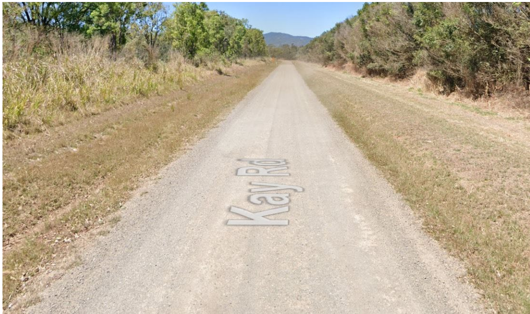
Photograph 2.26 – Kay Road Chainage 3600
