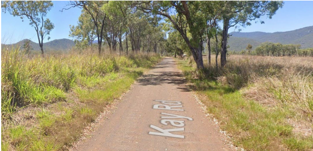
Photograph 2.31 –Kay Road Chainage 5400
