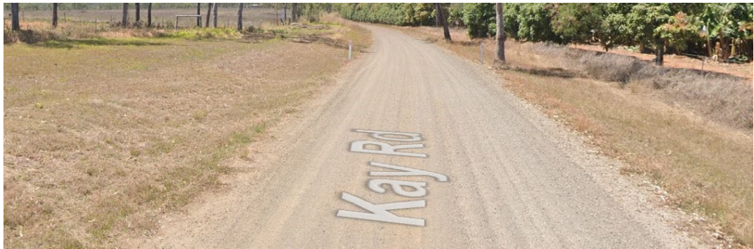
Photograph 2.29 – Kay Road Chainage 4850
