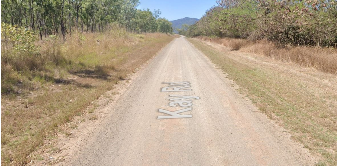
Photograph 2.28 – Kay Road Chainage 4200
