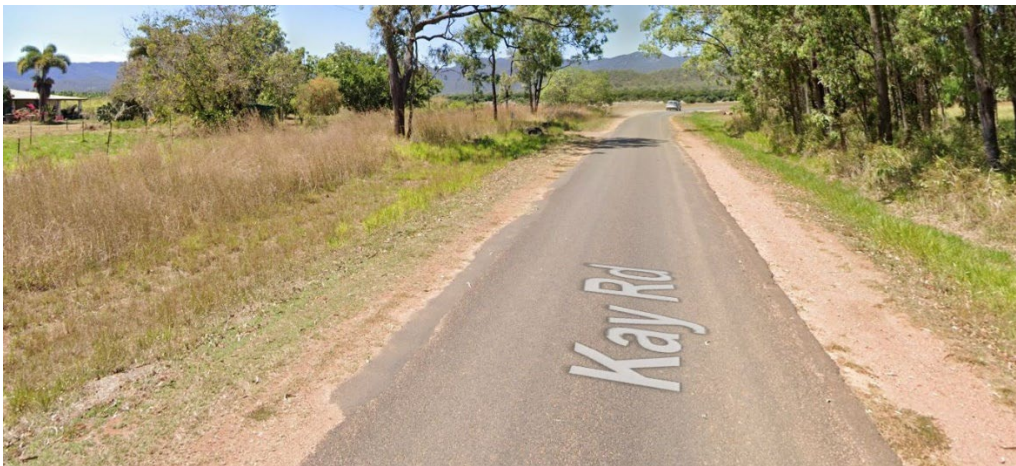
Photograph 2.23 – Kay Road Chainage 2400
