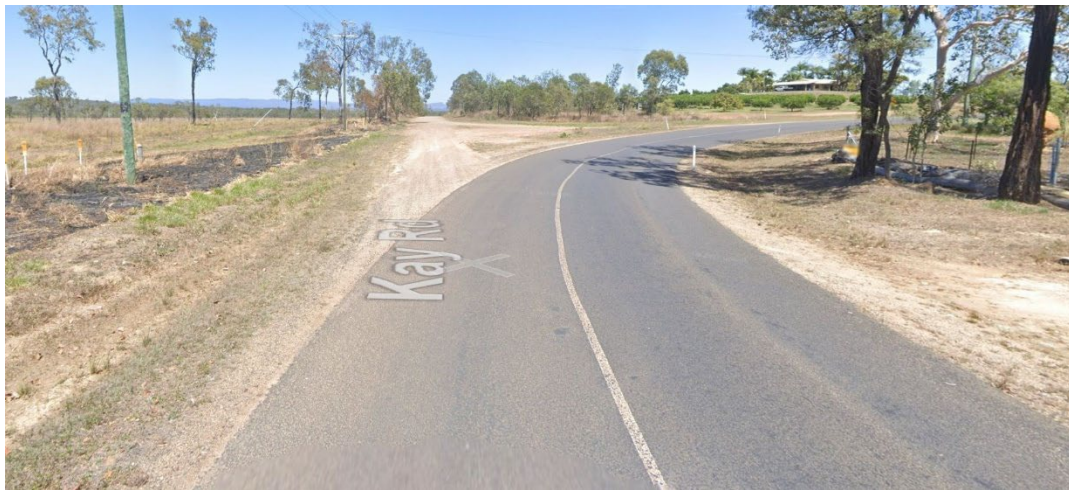
Photograph 2.20 – Kay Road Chainage 1550
