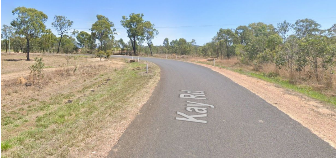
Photograph 2.19 – Kay Road Chainage 1300
