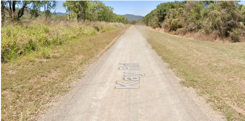
Photograph 2.25 – Kay Road Chainage 3400
