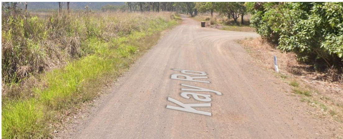
Photograph 2.30 – Kay Road Chainage 5250
