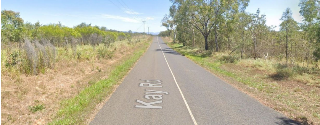
Photograph 2.22 – Kay Road Chainage 2100
