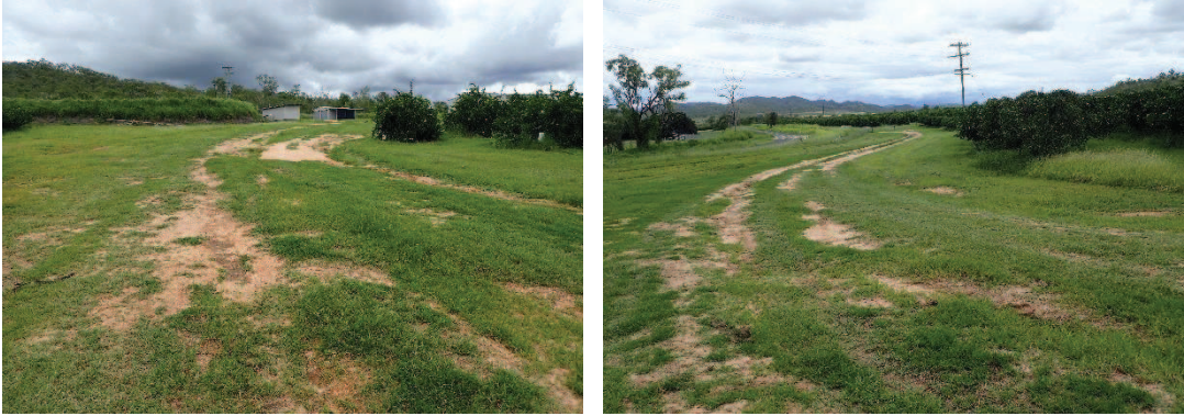
Plate 3: Photographs of mapped drainage features intersecting the access track in the Lot
