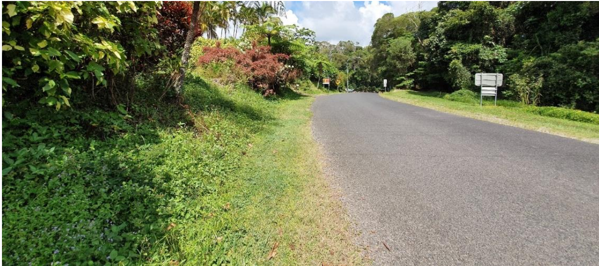
Figure 4: Photograph of one-way crossfall with limited table drain capacity (approximately CH90)
