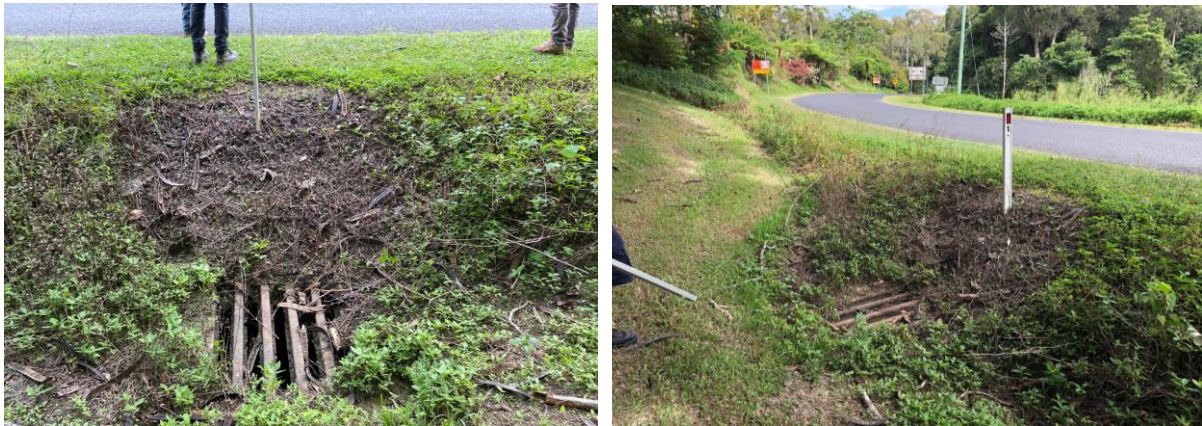
Figure 2: a) Existing Inlet pit to Black Mountain Road cross culvert to be upgraded due to nonstandard arrangements. b) Existing table drain directing water into inlet pit.
