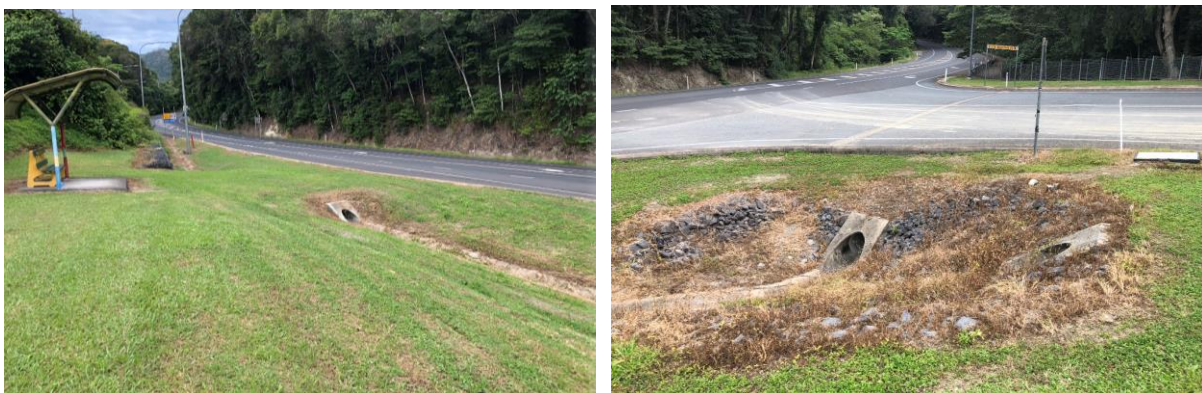
Figure 3: a) culvert allowing access to bus stop with Kennedy Highway in background. b) Culvert directing water from site under black mountain road into tributary of Barron River and culvert conveying water captured in table drain along south western road frontage of proposed development site.
