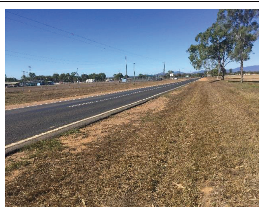
Mareeba Dimbulah Road table drain fronting site (looking east)
