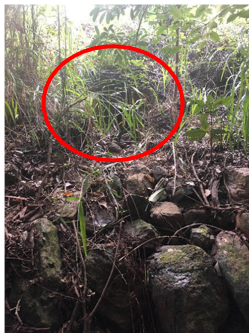
Image 6 – Existing rock batter protection at outlet (headwall circled in red)
