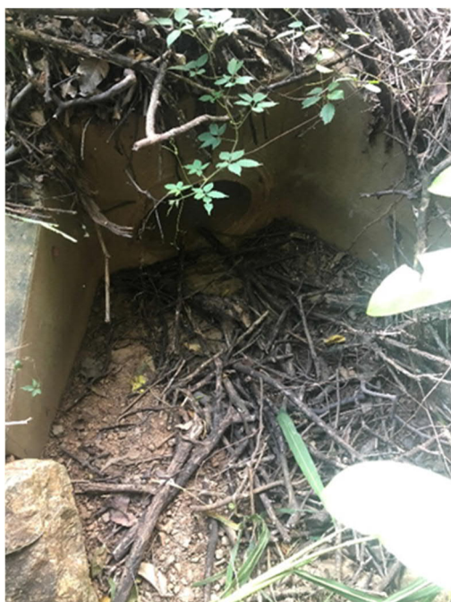
Image 5 – Existing headwall outlet from kerb inlet pit on Masons Road
