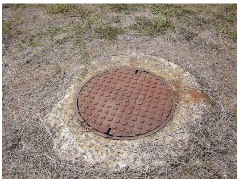
Photograph 8.2 – Existing Sewer Manhole within Site
