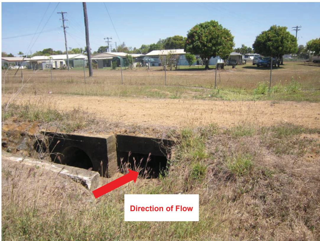
Photograph 5.5 – Cross Culverts Under Abandoned Rail Formation
