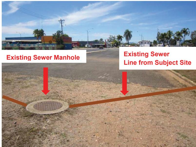
**Photograph 8.3 – Existing Sewer Manhole in Rankin Street**
