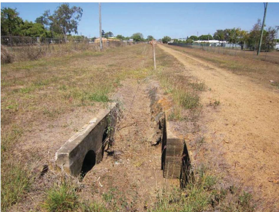
**Photograph 2.8 – Culverts Under Rail Formation**
