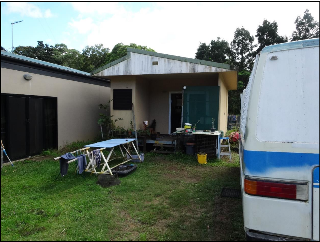
Photo 9: Detail of unserviced 'sleepout'
