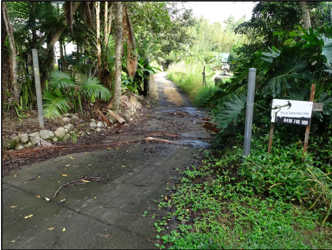
Photo 2: Existing driveway to proposed Lot 102.
