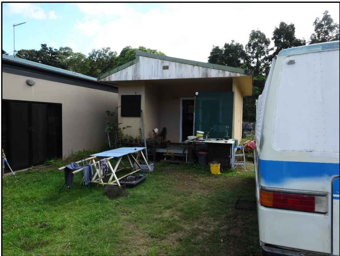
Photo 9: Detail of unserviced 'sleepout'
