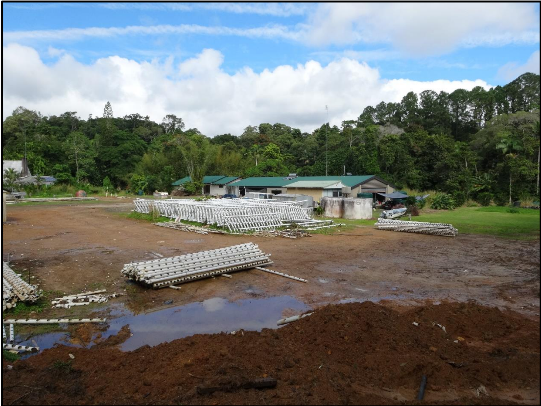
Photo 6: View across site from northeast corner
