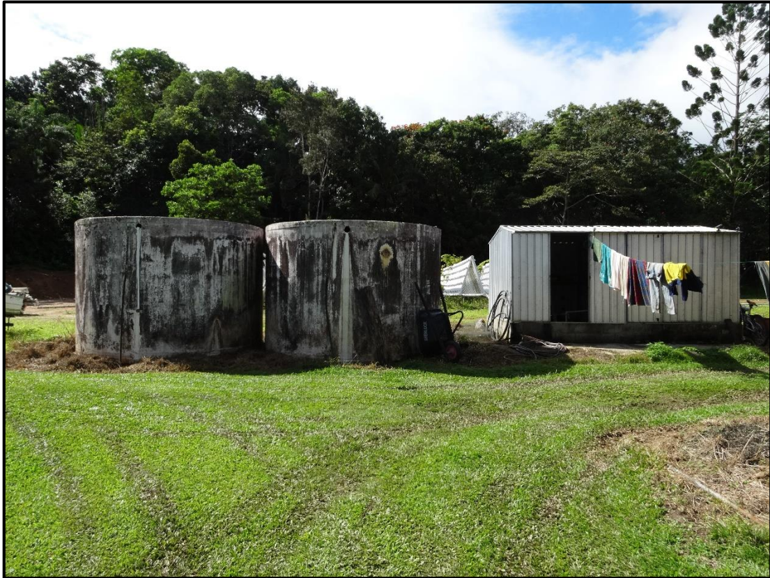
Photo 10: Detail of water tanks and pump shed
