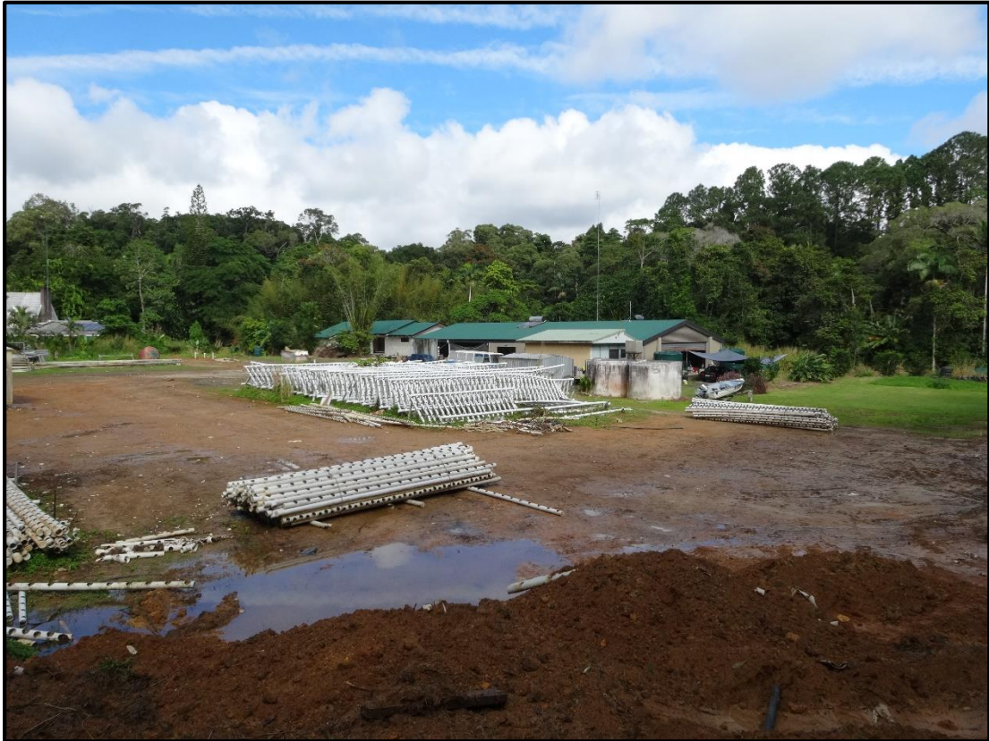
Photo 6: View across site from northeast corner
