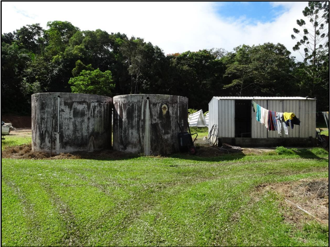
Photo 10: Detail of water tanks and pump shed
