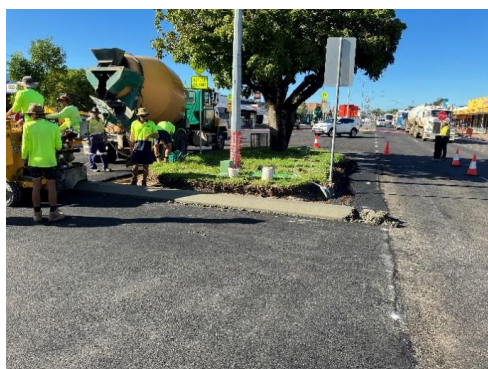
Installation of maintenance kerbing
