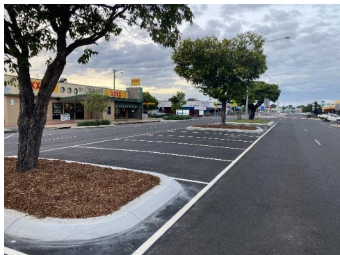
Completed Line Marking
