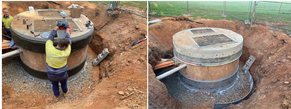
Installation of support rings and epoxy resin
