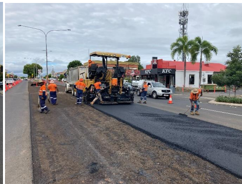
Placement of DG10 asphalt overlay
