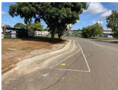
Completed node opposite PIMS
