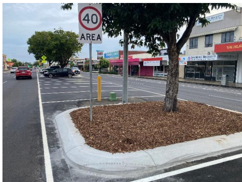
Completed Line Marking
