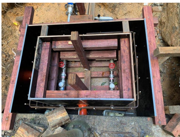
New discharge pipework assembly into the pump station and concrete encased housing
