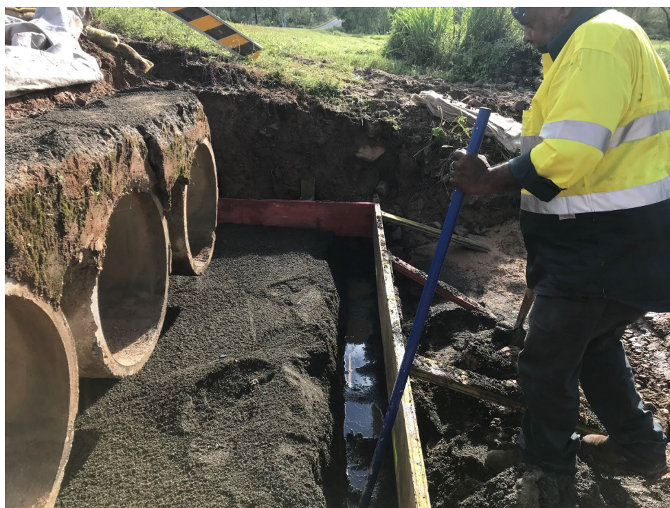
Photo 4 Wolfram Road Bitumen Seal Widening Safety Upgrade
