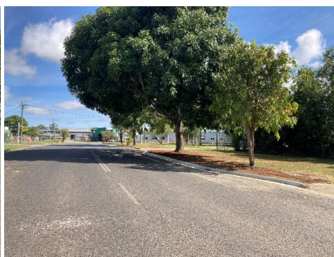
Completed node opposite Mareeba Workers Club
