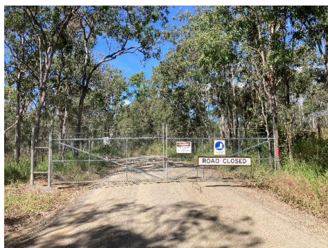
Davies Creek Road closure
