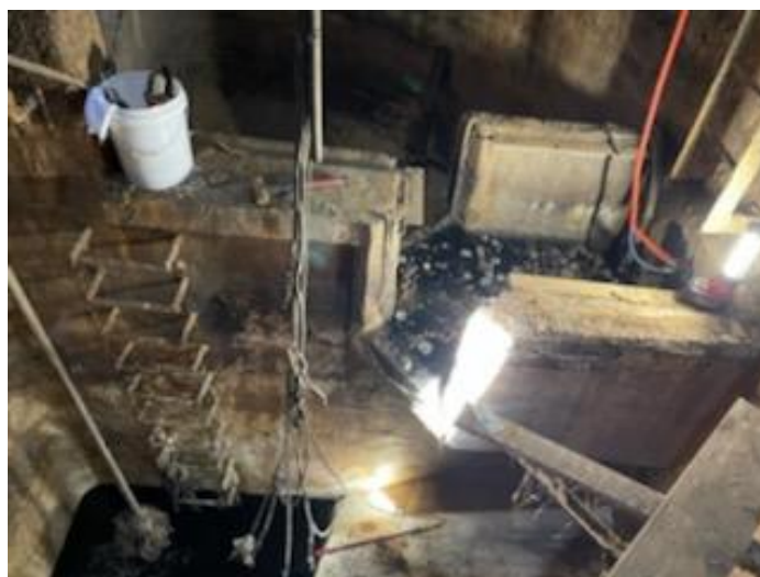
Demolition of the upper pump station structures and internal pump station stripped out
