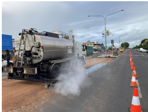
Application of 7mm primer seal
