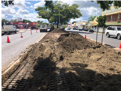
Preparation of new northern median garden bed
