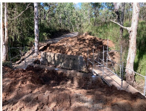
Scaffold & exposed bridge abutments
