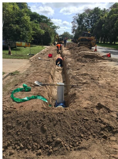
Installations of the new 300mm diameter PVC Supermain along Moody Street
