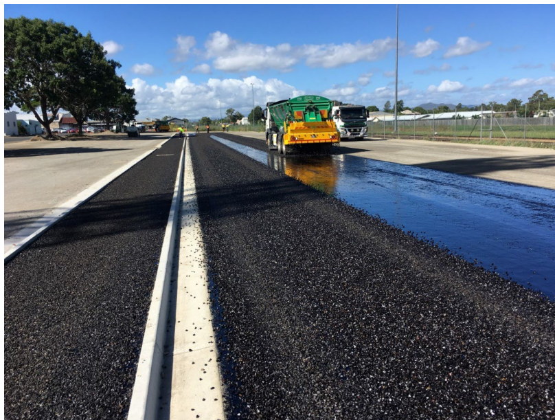
Photo 2 Railway Avenue CBD Car Park Upgrade.
