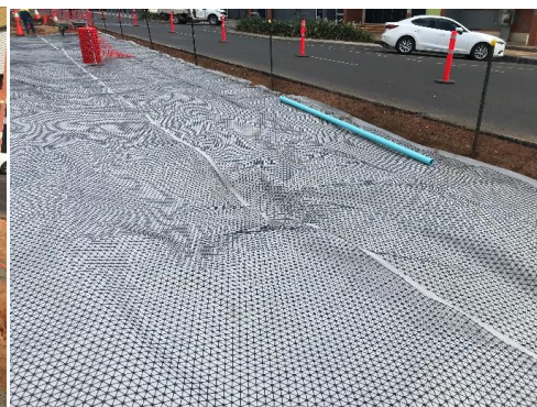
Geofabric covering replaced unsuitable material
