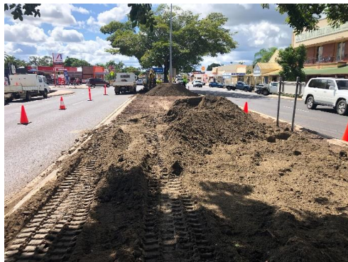
Preparation of new northern median garden bed
