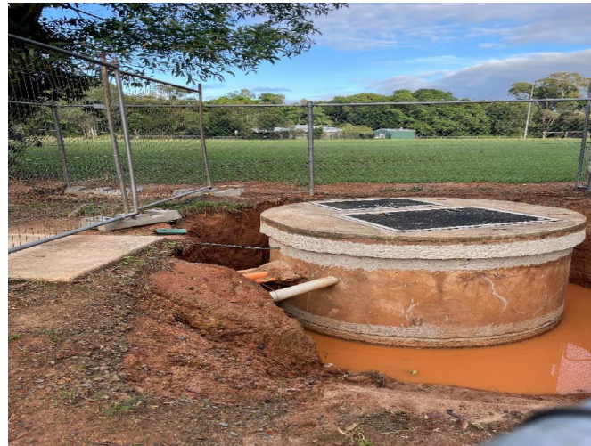
Site excavated to install root barrier
