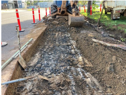
Removal of failed pavement & damaged K&C
