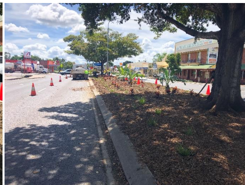
Planting out new northern median garden bed
