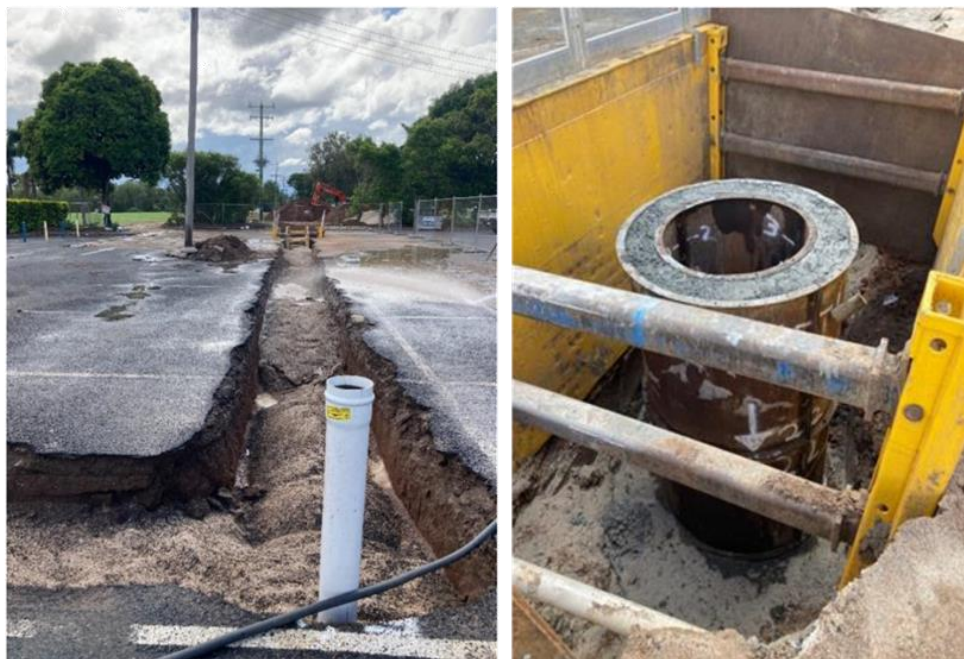
Connection of the Hub Complex to the new gravity sewer main underway
