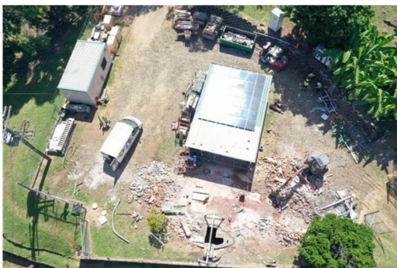
Demolition of the upper pump station structures
