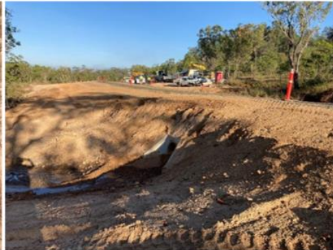
Repaired Sunken Culvert
