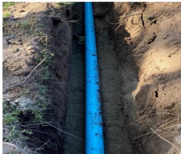
Installations of the new 100mm diameter PVC Supermain water main Hampe Street
