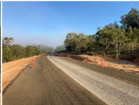
New Material installed on Shoulder
