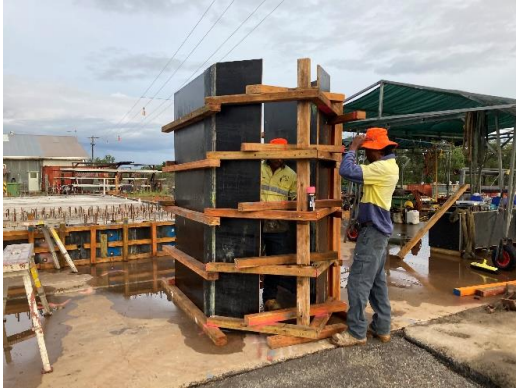
Preparing formwork for pier extension
