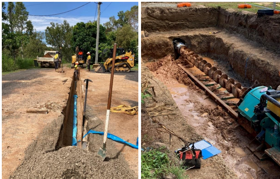
Installations of the new 100mm diameter PVC Supermain water main Starcke Street and under boring from the cemetery entrance under Vaughan Street
