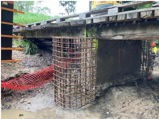
Pier reinforcement in place
