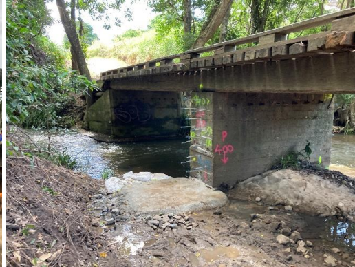
Pier dowels installed
