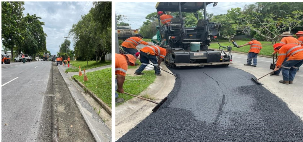
Road reinstatement over the water main installation
