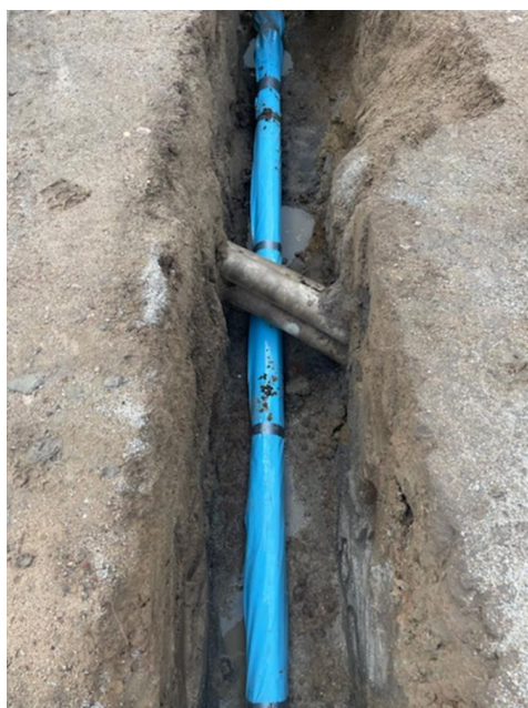
Installations of the new 100mm diameter PVC Supermain water main Starcke Street
