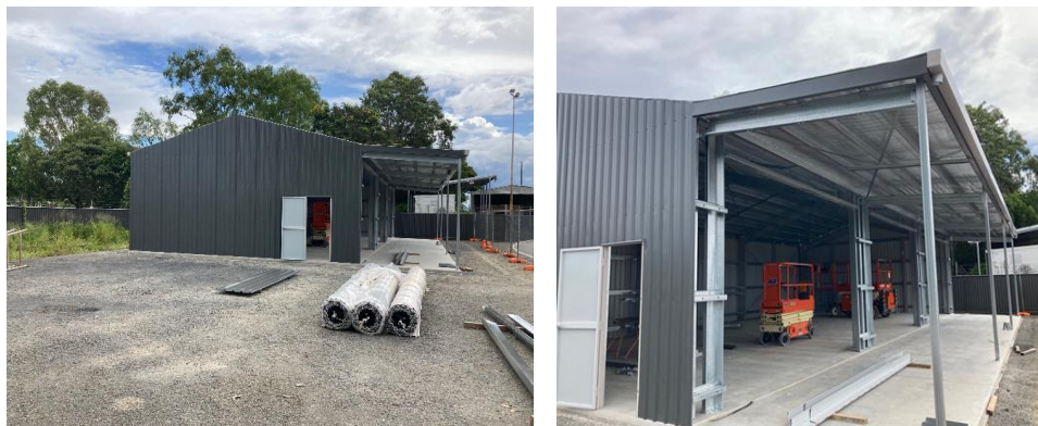
New Buy Back Shop Shed under construction
