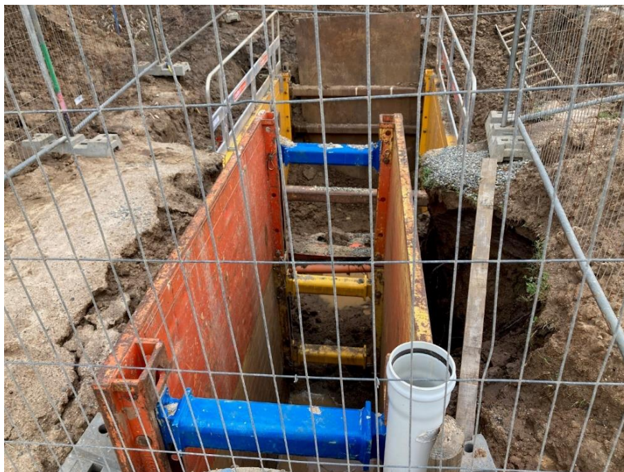
Excavation works for gravity sewer main
