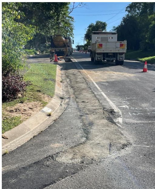
Laying and installation of the new 150mm diameter PVC Supermain water main
