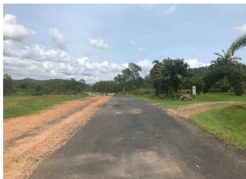
Pavement failure at Ch 7960
