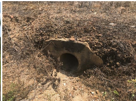
Narrow culvert and failing headwall Ch 8600
