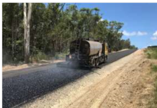
Bitumen Sealing (2 nd Coat)
