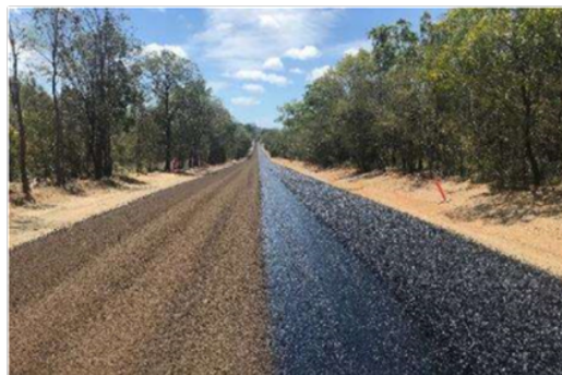
Bitumen sealing (2 nd coat)
