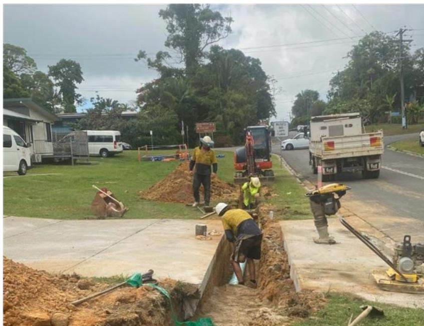
*Laying and installation of the new 150mm diameter PVC Supermain water main west of Thongon St intersection*
