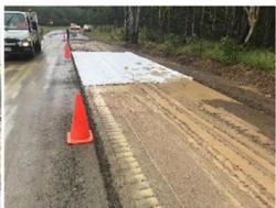
Geofabric put in place due to unsuitable subgrade
