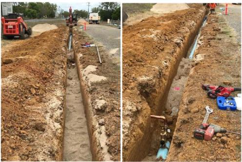
Laying and installation of the new 150mm diameter PVC Supermain water main
