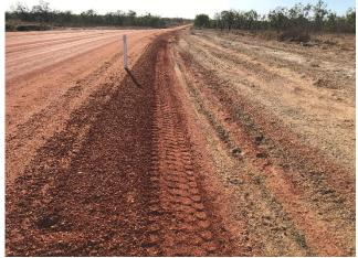
Completed running surface and table drain
