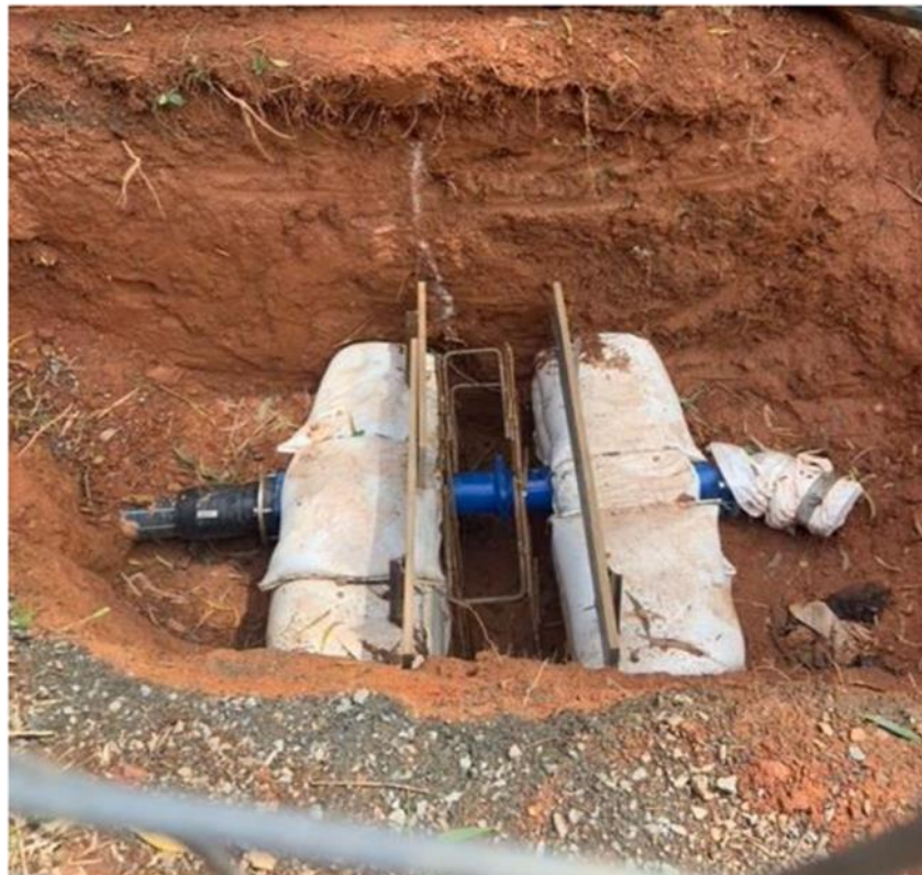
Cut in and laying new discharge and suction lines to the new booster pump station
