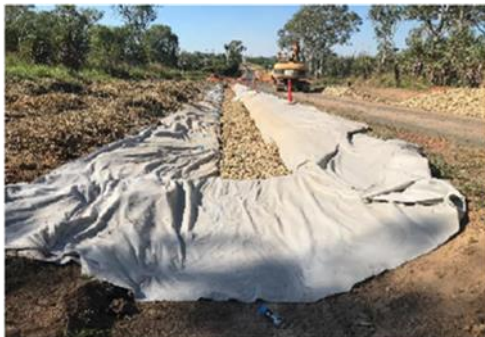
Replacing unsuitable material with rock and bitumen
