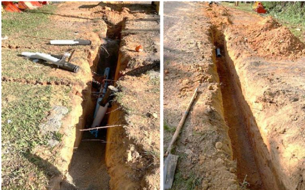
Newly pipeline construction and service connections
