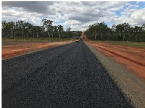
Sealing between McBean Road and causeway
