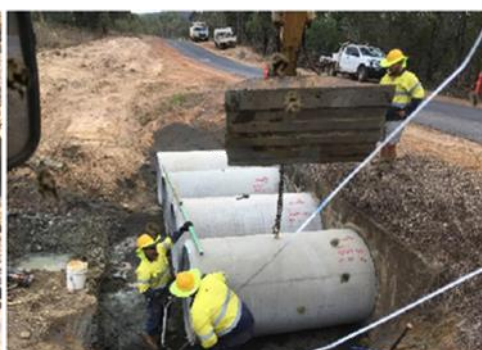
Installing RCP extensions
