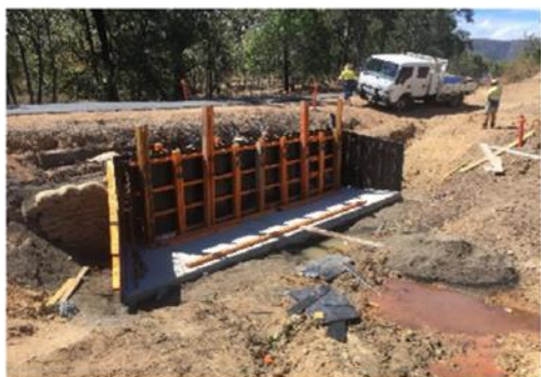
New headwall formwork
