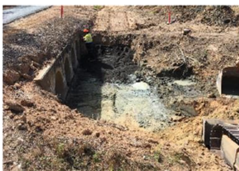
Preparation form major culvert extension
