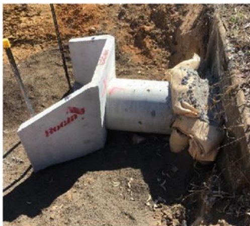
Existing culvert extension
