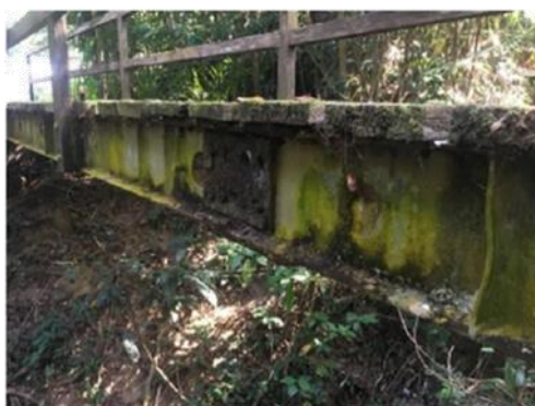
Old Barang St Pedestrian Bridge - corrosion
