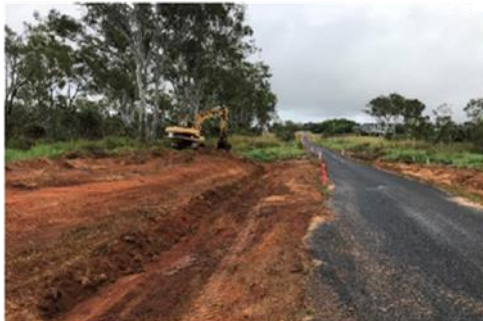
Drainage works at causeway site
