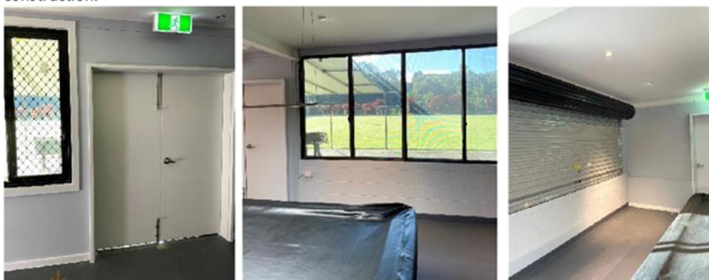
Ground floor: Refurbishments undertaken to including waterproofing, new fire doors and roller doors
