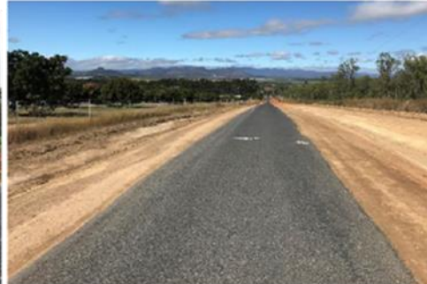
Completed subgrade between McBean & Stanton Roads
