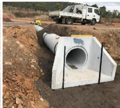
Newly installed culvert
