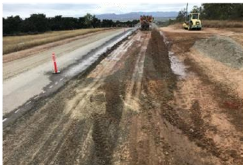
Installation of base gravel in widening
