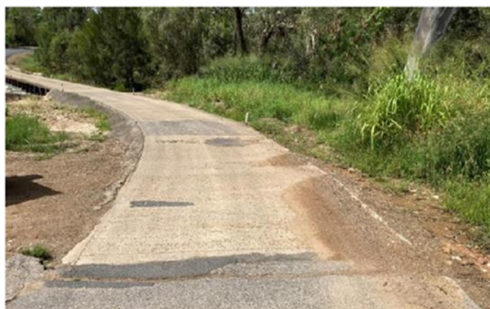
South western end of culvert (before)
