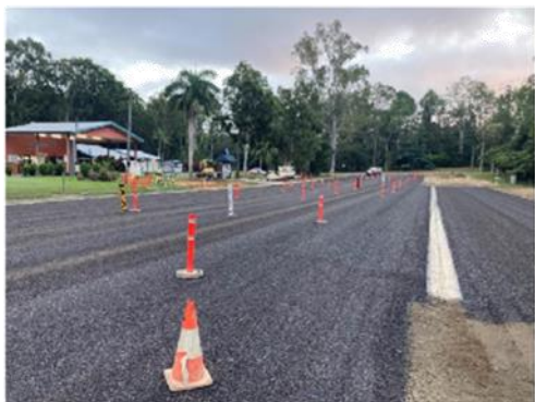
Completed sealed pavement
