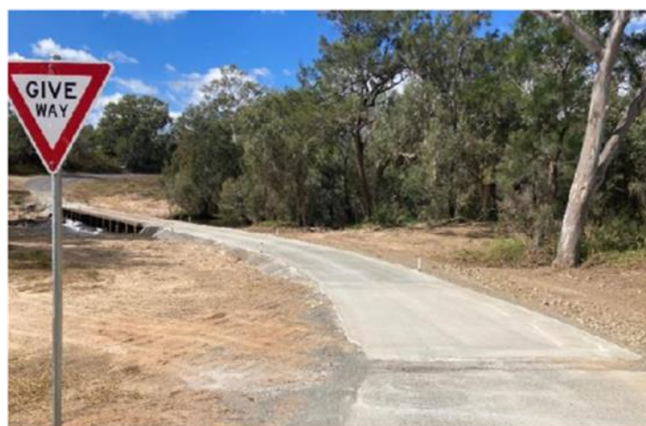
South western end of culvert (after)
