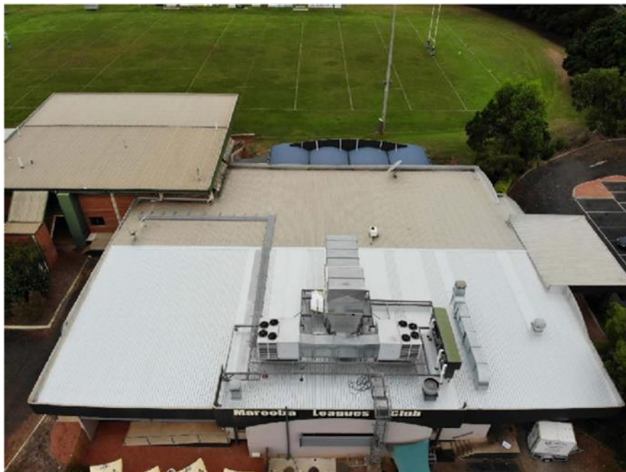
Completed works seen from a drone perspective
