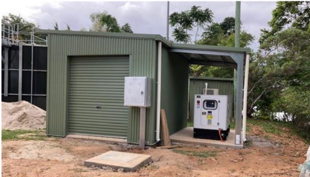
Booster station shed and standby generator
