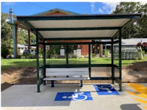
Completed bus shelter
