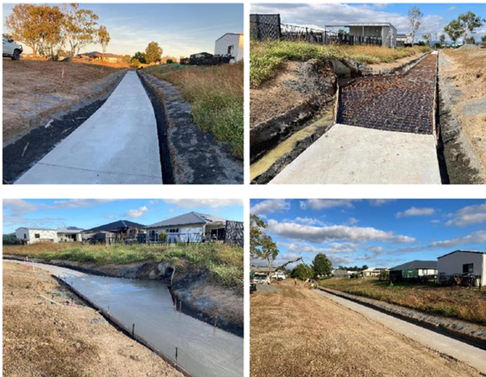
Construction of concrete invert
