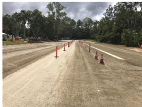
Completed unsealed pavement
