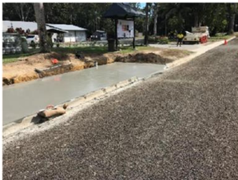
Bus shelter slab
