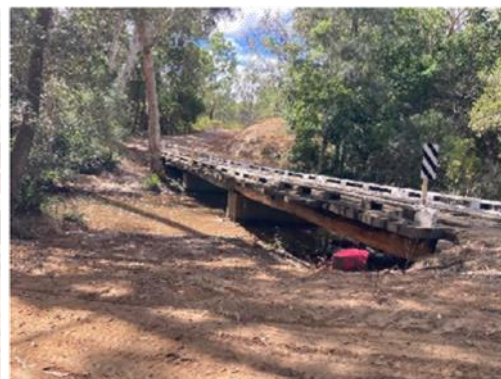
Completed bridge works
