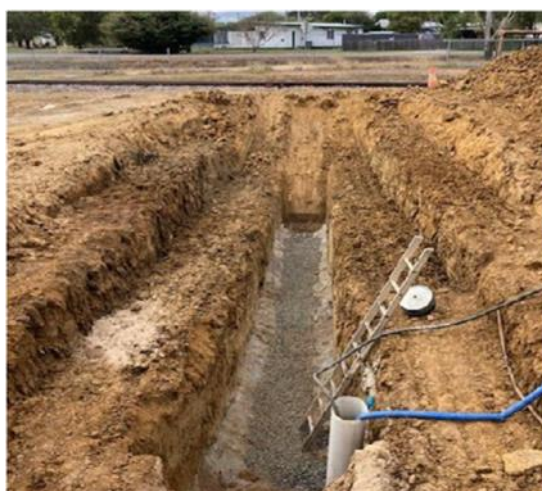
Excavation works to install the section of sewer main under the rail line
