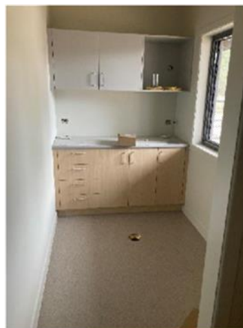
Internal kitchen fit-out with vinyl sheet flooring
