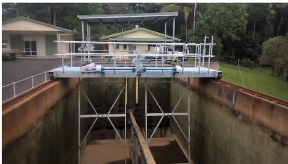
Clarifier trolley assembly
