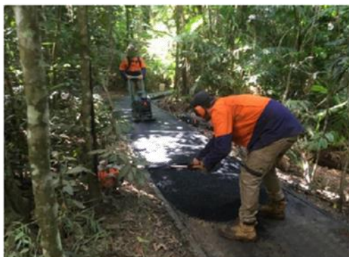
Jungle Walk - asphalt resurfacing
