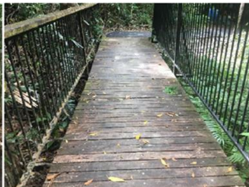
Jungle Walk - Bridge 1 old deck boards
