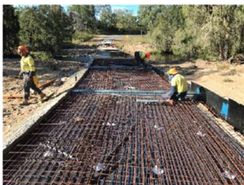
Steel reinforcing placement
