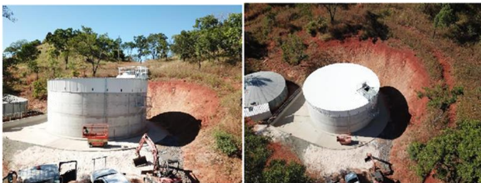
Newly constructed concrete reservoir with roofing structure construction
