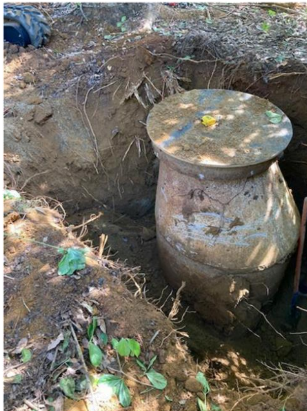
Excavation around manhole to remove tree root intrusions and sealing of concrete joints
