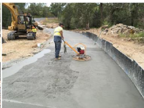
Finishing concrete topping slabs
