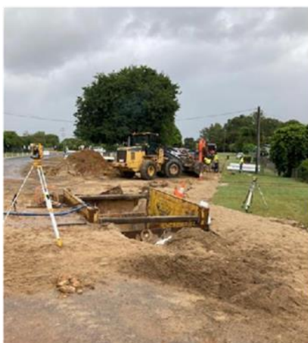
Excavation works and manhole construction Strattmann Street
