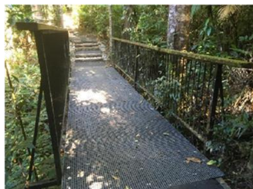
Jungle Walk - Bridge 1 New FRP Deck
