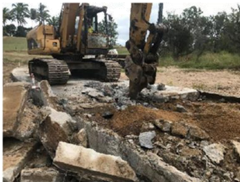
Removal of damaged and cracked topping slabs
